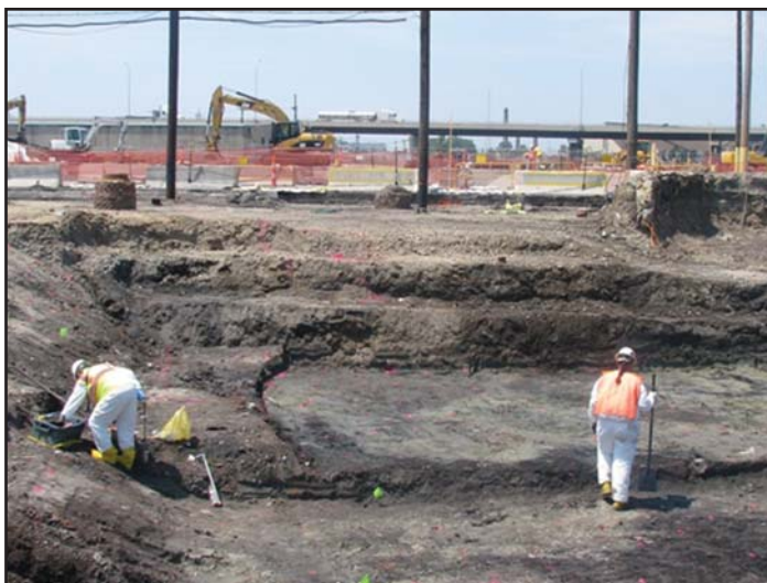
St. Louis Downtown Site - Plant 7 - 700 Pad Excavation
