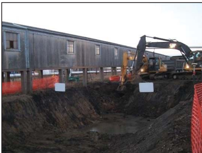
Iowa Army Ammunitions Plant - Line 1 Excavation
