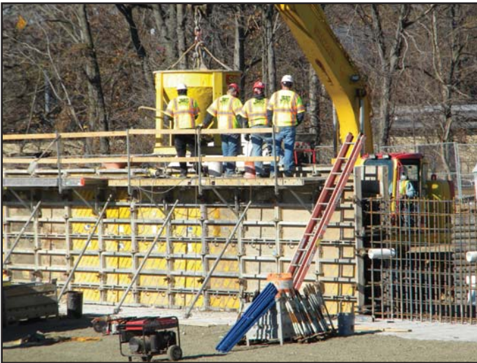
Maywood Site - Concrete placement for loadout pad retaining wall
