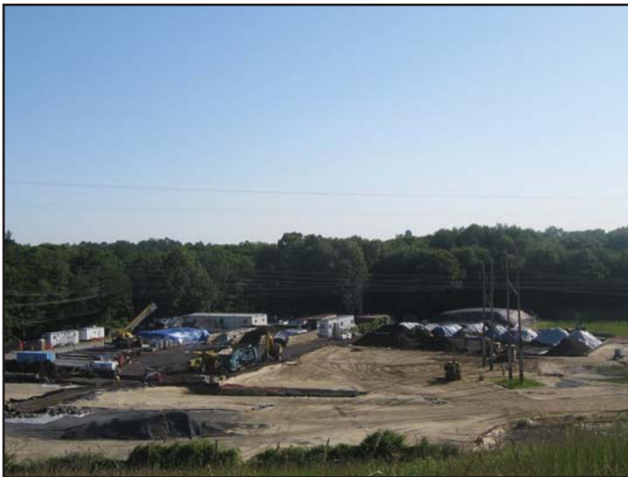
FUSRAP cleanup at the Shpack Landfill Site
