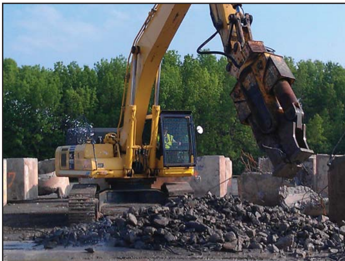
Linde Site - Processing decontaminated tunnel sections for recycling
