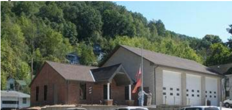
New facility by relocations contract
