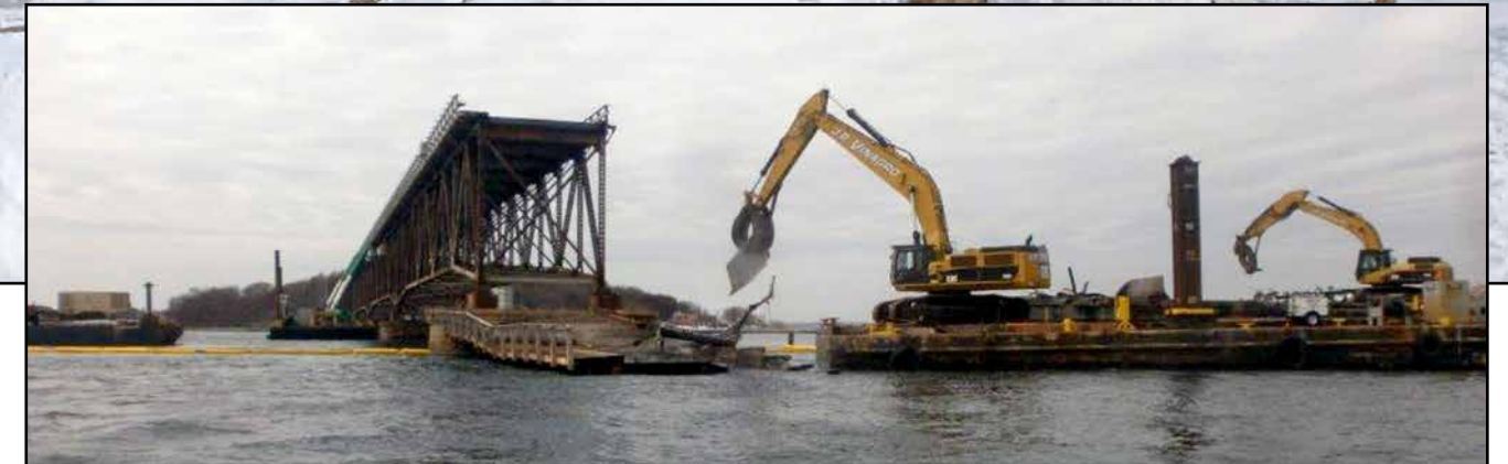
ABOVE: A view of the Long Island Bridge in Boston Harbor prior to demolition. (Photo by Paul Sneeringer) RIGHT: Demolition contractor Walsh Construction removes and sorts bridge debris with barges and excavators. (Photo courtesy Walsh Construction)
