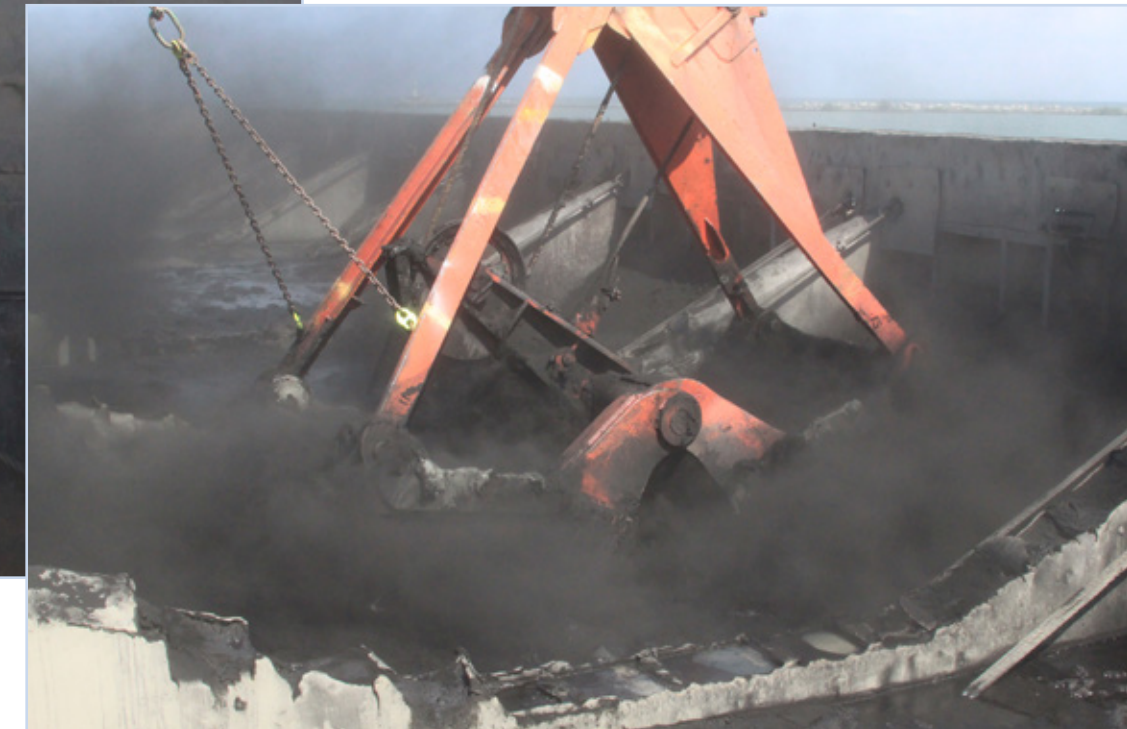
Super sacks of powdered and granular activated carbon are added to a scow of dredged sediment before mixing with a clamshell bucket. A clamshell is used to thoroughly mix activated carbon and dredged sediments in a scow, before it is placed in the open lake. (Courtesy photos)
