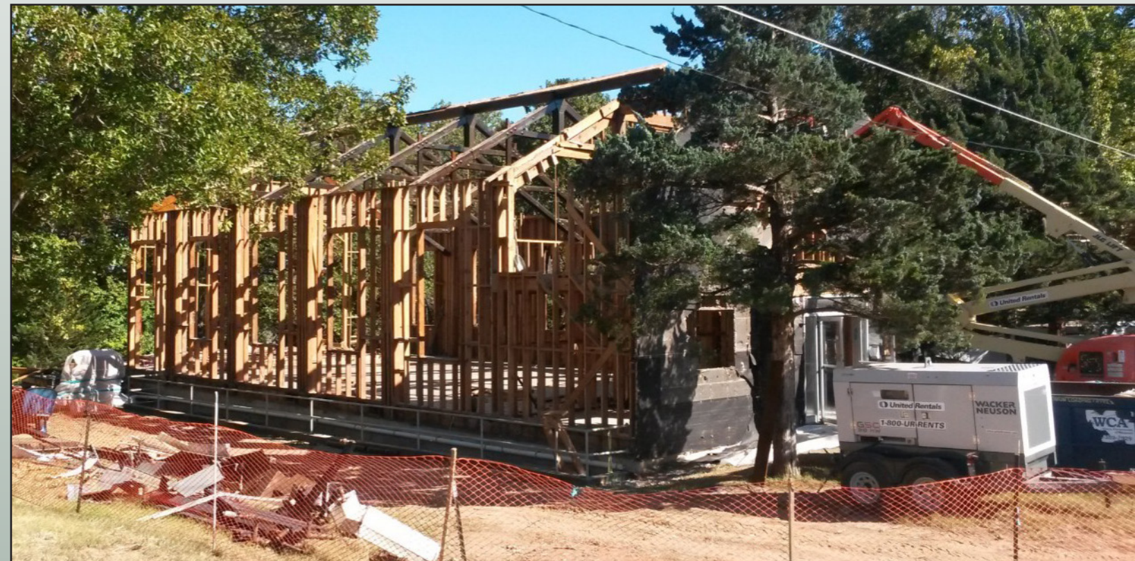
LEFT: Bhate employees work to deconstruct a chapel — one of three World War II era buildings selected for the deconstruction pilot program — on Fort Leonard Wood, Missouri. BELOW: Deconstruction of the chapel began Sept. 16, with major deconstruction completed by Oct. 7. Once the building was removed, the contractors backfilled and seeded the lot. Overall, 252 tons, almost 85 percent of the material collected from the chapel was recycled or reused. (Courtesy photos)
