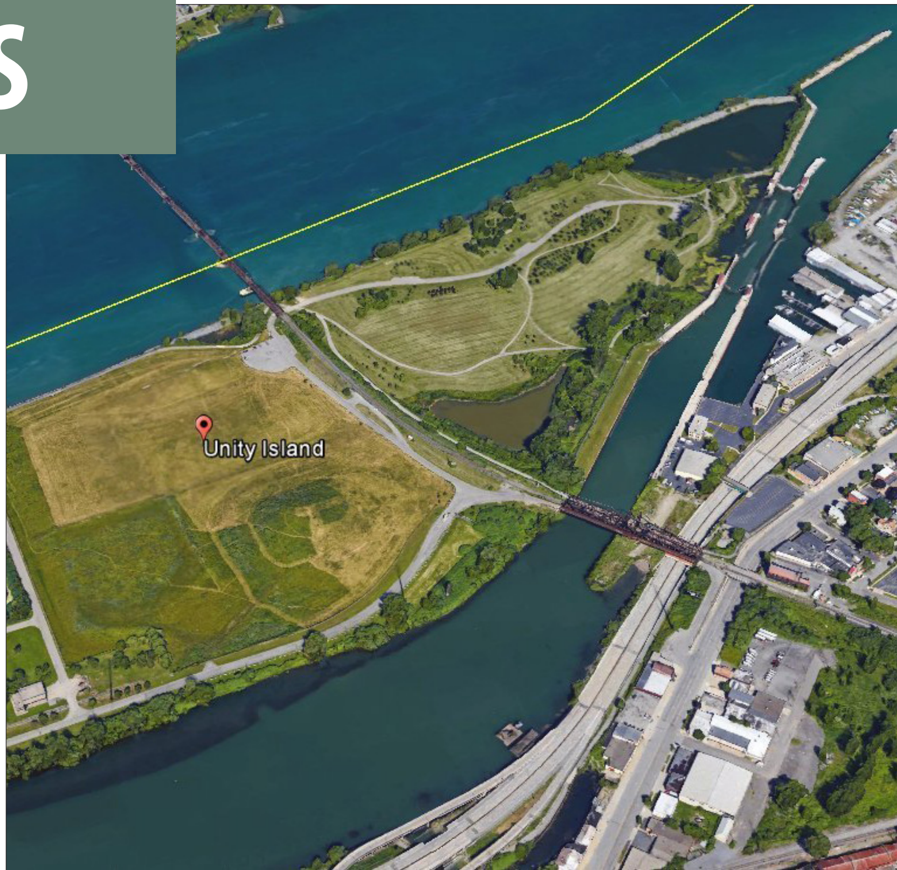
The U.S. Army Corps of Engineers Buffalo District awarded a $1.39 million contract in September to Tidewater Inc. of Elkridge, Maryland, in support of the Unity Island Aquatic and Riparian Invasive Species Management and Habitat Restoration Project for the removal of aquatic invasive species (AIS) from Unity Island in Buffalo, New York. As part of the Great Lakes Restoration Initiative, the demonstration project will be conducted in coordination with the city of Buffalo and the Engineer Research and Development Center. Methods used to control AIS will be monitored for a period of three years before potentially being employed throughout the Great Lakes in coastal wetland environments similar to Unity Island. The project includes implementing AIS control and management, introducing container-grown woody, shrub and herbaceous native plant species, planting in-water submerged aquatic vegetation (SAV), installing in-water fish attraction structures, planting in-channel SAV and installing fish attraction structures, and expanding riparian and wetland buffers. The goal of this demonstration is to evaluate the efficacy of a number of invasive species removal methodologies. (Photo by Andrew Kornacki)
