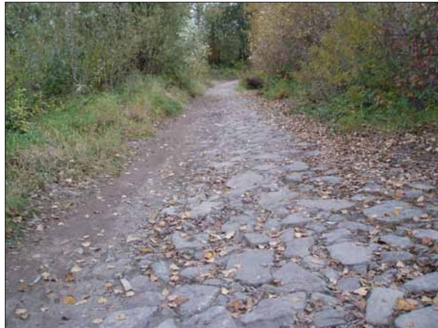
A 1930s-era dam constructed across the East Channel of the Sandy River was removed by the Corps of Engineers September 2013 during a habitat restoration project. Since its construction, sediment settled around the dam until it appeared to be a stone-filled path.
