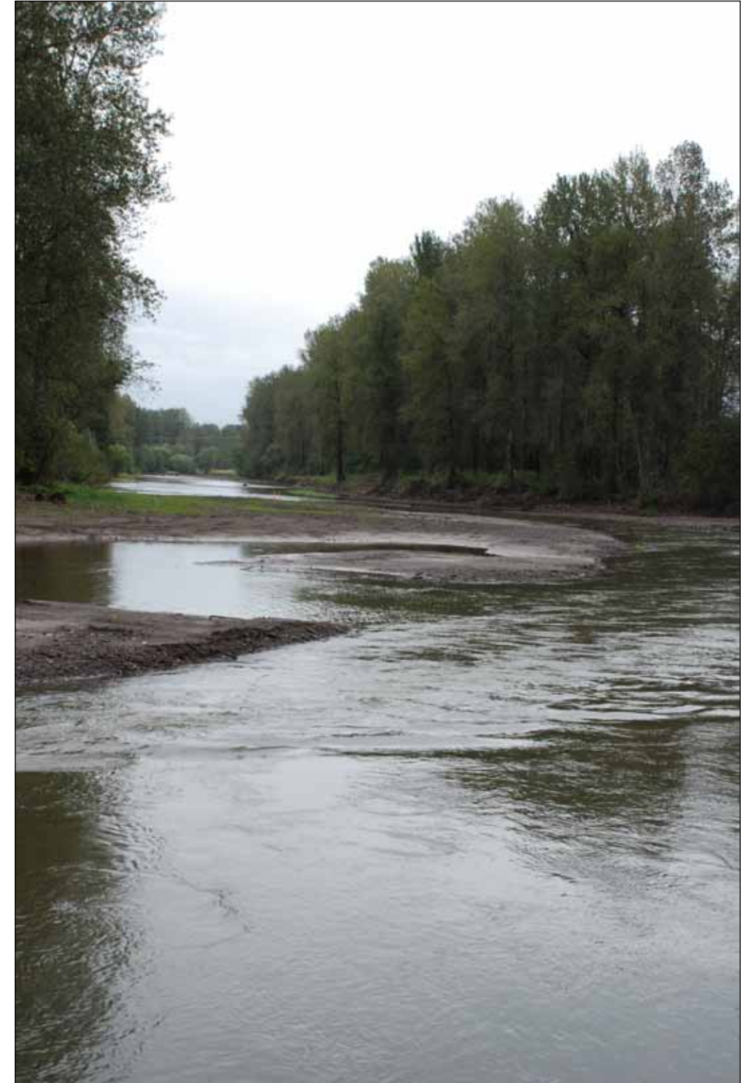
The East Channel of the Sandy River flows freely after Corps contractor LKE removed a 1930s-era dam. The restoration of flow will provide healthy habitat for young fish as the delta returns to a natural, braided river environment.
