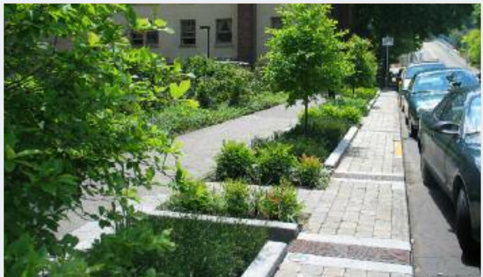
Green Street projects currently retain and infiltrate 36.9 million gallons of stormwater per year and have the potential to manage 7.9 billion gallons.
