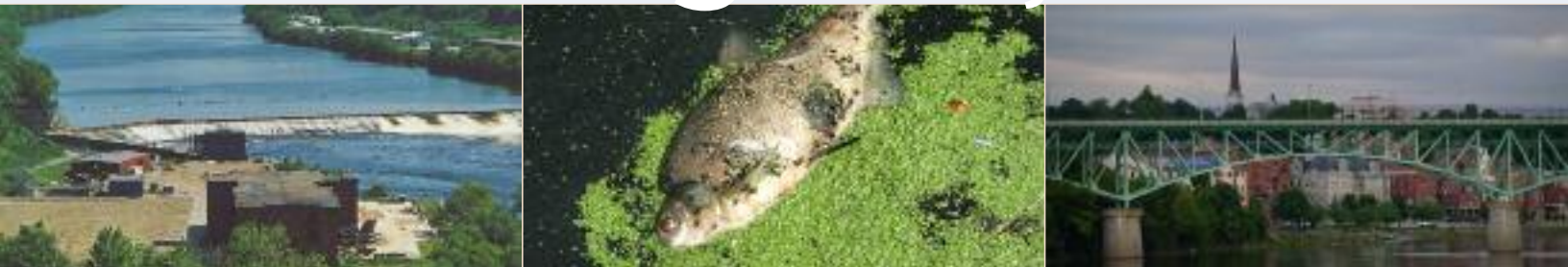
Left: Edwards Dam on the Kennebec River at Augusta before dam removal. Middle: The Edwards Dam and poor water quality decimated fish populations. Right: Augusta turned its back on the degraded river.
