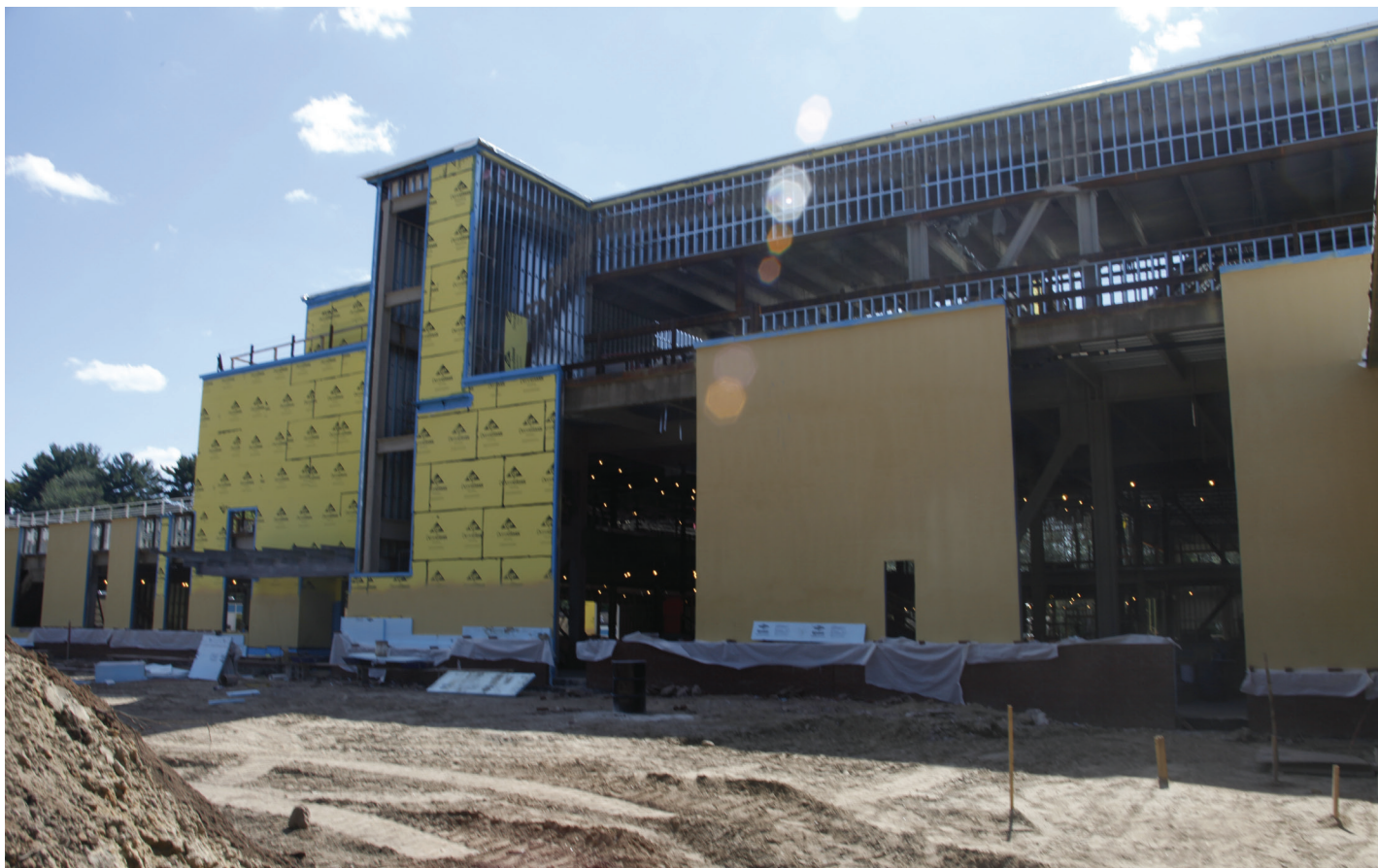
Hanscom Middle School construction on Hanscom Air Force Base, Massachusetts.
