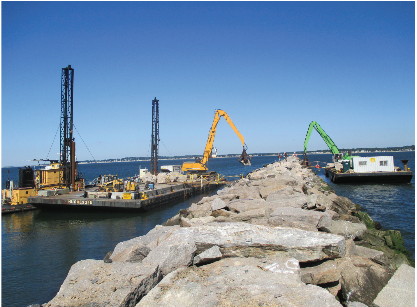
District contractor Mohawk Northeast performs breakwater repairs at New Haven Harbor.
