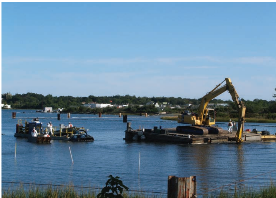
Work at the New Bedford Superfund Site.
