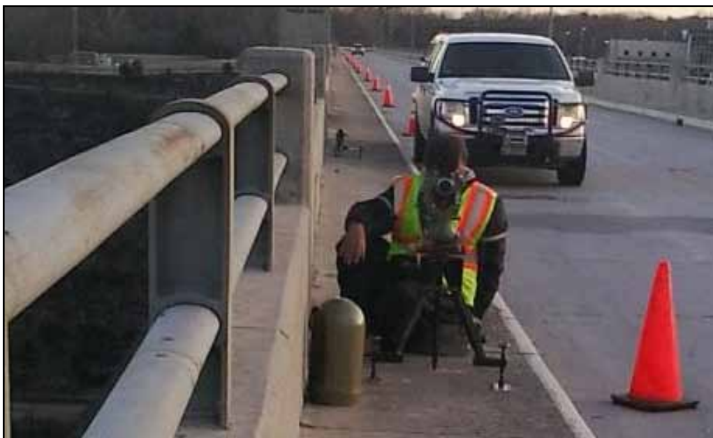
Photo by Robert Meyer Robert Dudley of the Little Rock District sets up on an Arkansas bridge for an evening of dam alignment surveying at Table Rock Dam, Branson, Mo.
