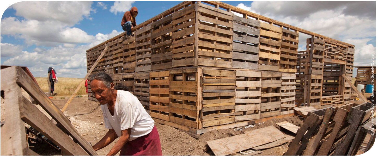
House being built on Pine Ridge Reservation
