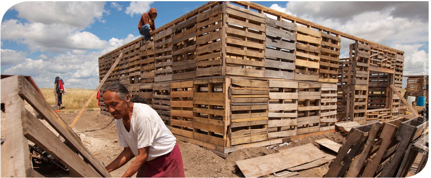
House being built on Pine Ridge Reservation
