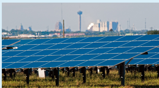
Figure 10.8. Photovoltaic panels convert sunlight directly into electricity. Utility-sized solar power plants require large tracts of land. Photo shows Duke Energy's 113-acre Blue Wing Solar Project in San Antonio, Texas, one of the largest photovoltaic solar farms in the country. (Photo credit: Duke Energy 2010 36 ).
