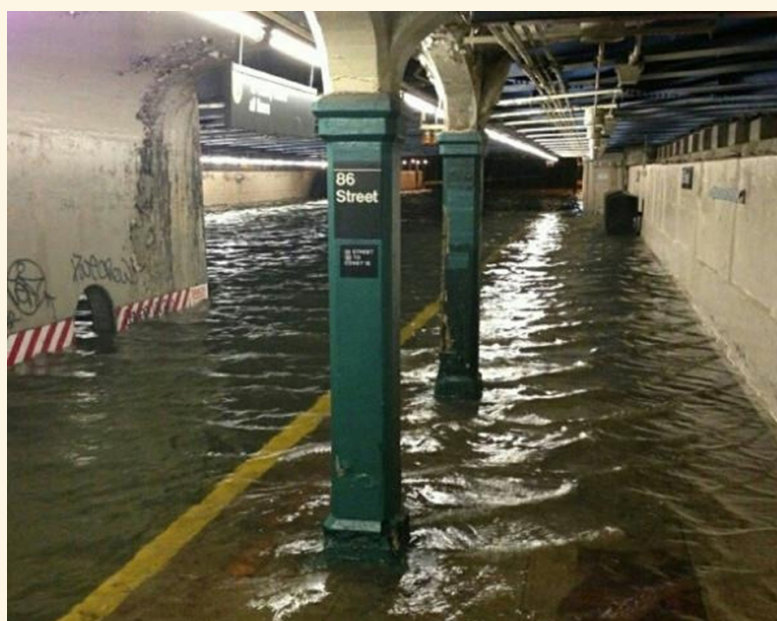
Figure 5.4. The nation’s busiest subway system sustained the worst damage in its 108 years of operation on October 29, 2012, as a result of Hurricane Sandy. Millions of people were left without service for at least one week after the storm, as the Metropolitan Transportation Authority rapidly worked to repair extensive flood damage (Photo credit: William Vantuono, Railway Age Magazine , 2012 46 ).
