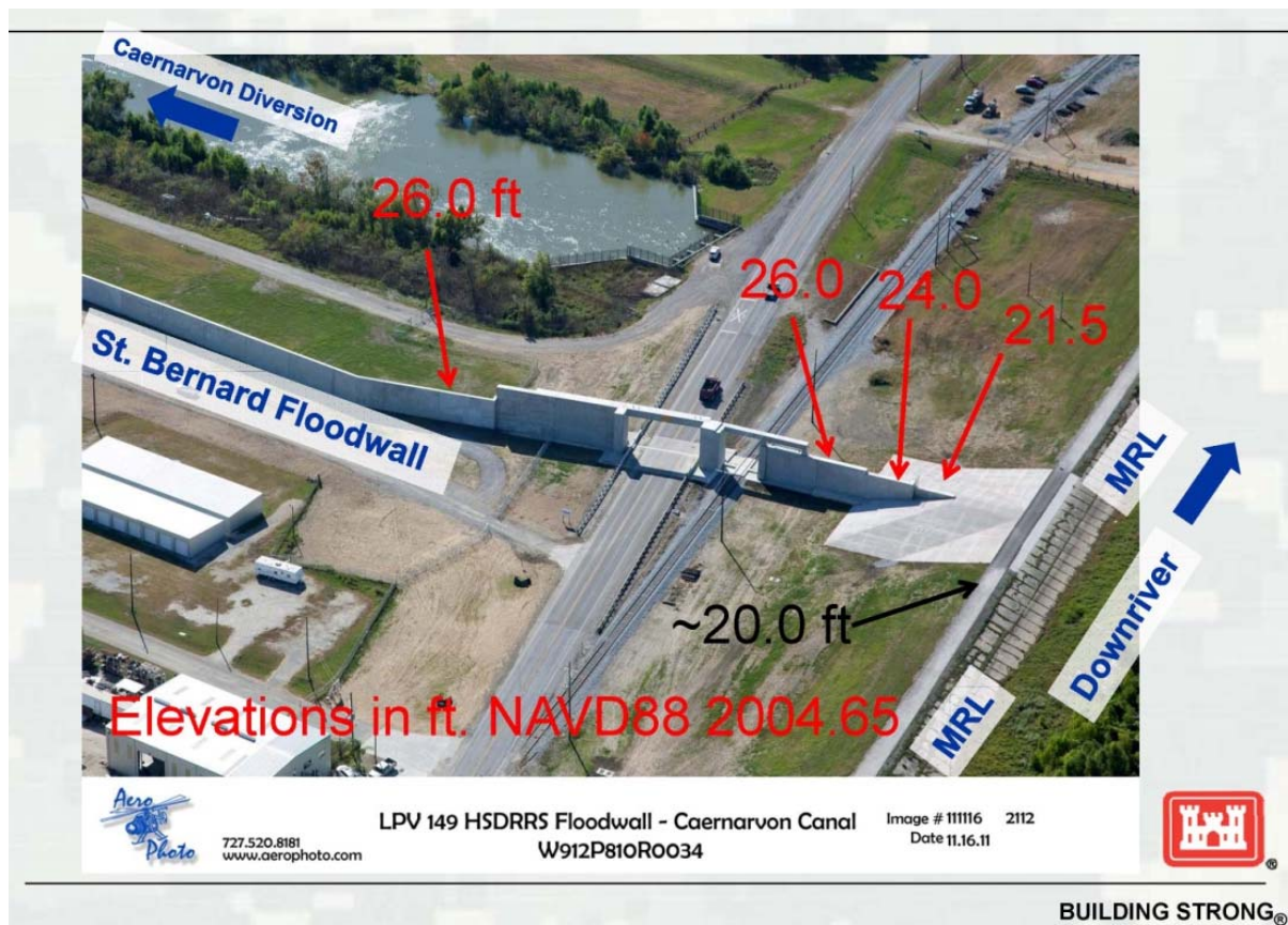
Figure 2 Aerial photo with structure elevations as built
