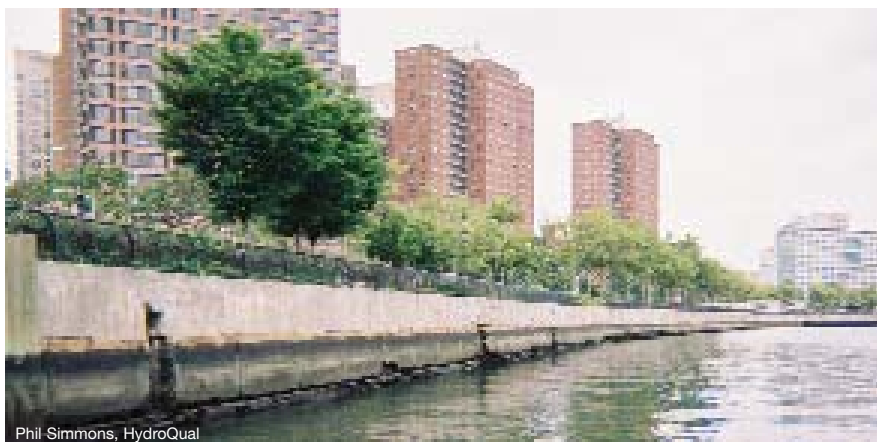
Sea level rise may warrant modifications to existing shoreline protective structures such as bulkheads and seawalls.
