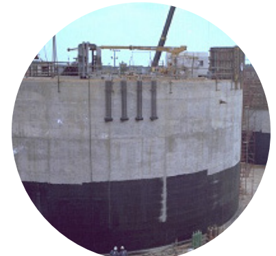
SRS waste tanks under construction
