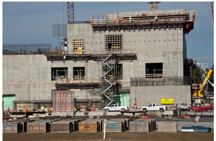
The Mixed Oxide Fuel Fabrication Facility began construction in 2007.
