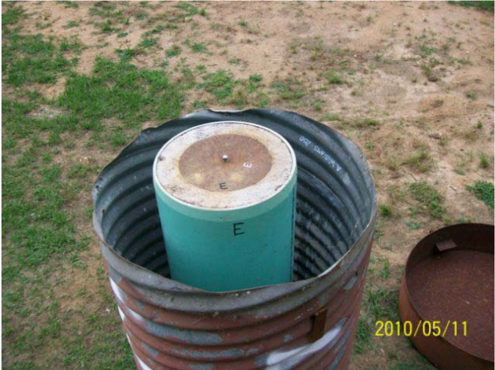
Figure 4-1c. Monument pedestal in soil (Savannah Bluff Lock and Dam – photo by Joyner Keeny, PLLC)
