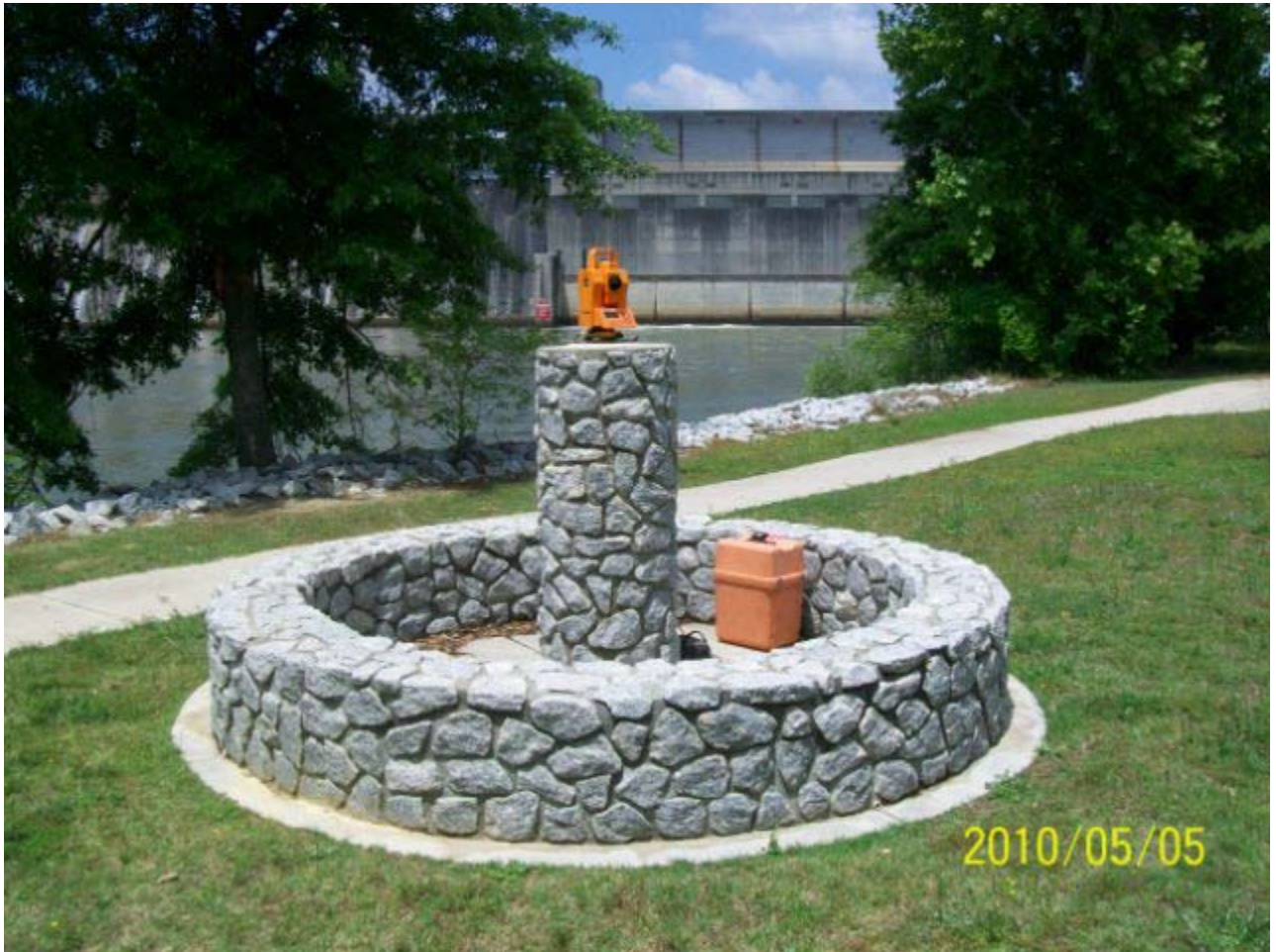
Figure 4-5. Pedestal monument at the Thurmond Dam used for structural deformation (Savannah District)
