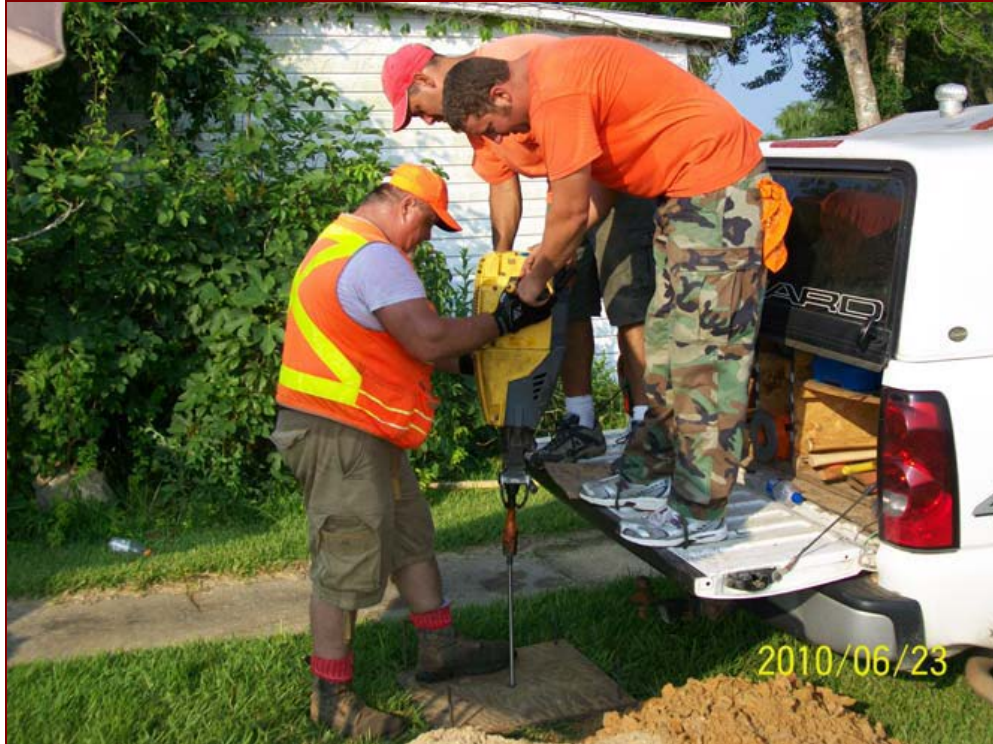
Figure 3-3. Driving a stainless steel rod with the Cobra Combi driving jackhammer Wilmington District (2010)
