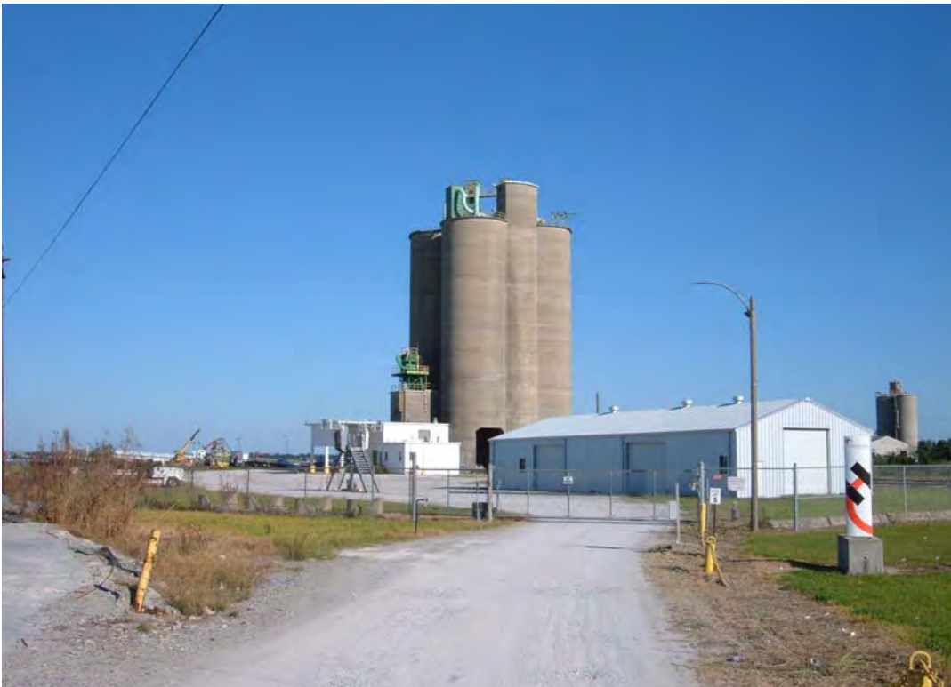
Photograph 4. View to southeast of Holcim facility on west channel bank.
