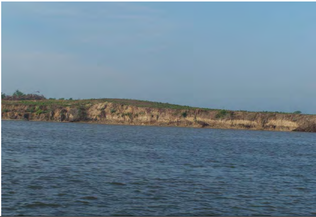
Photograph 21. View to west of channel bank near Hackberry showing erosion from vessel wakes.
