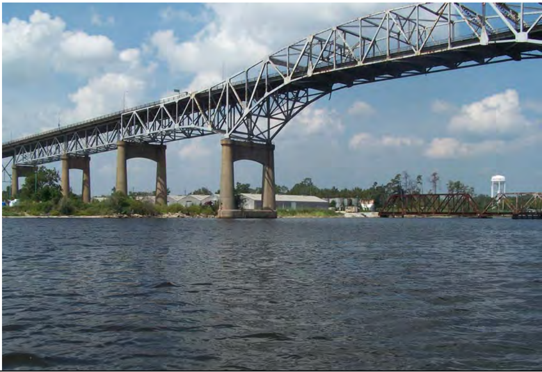
Photograph 1. View to north of channel near I-10 Bridge.
