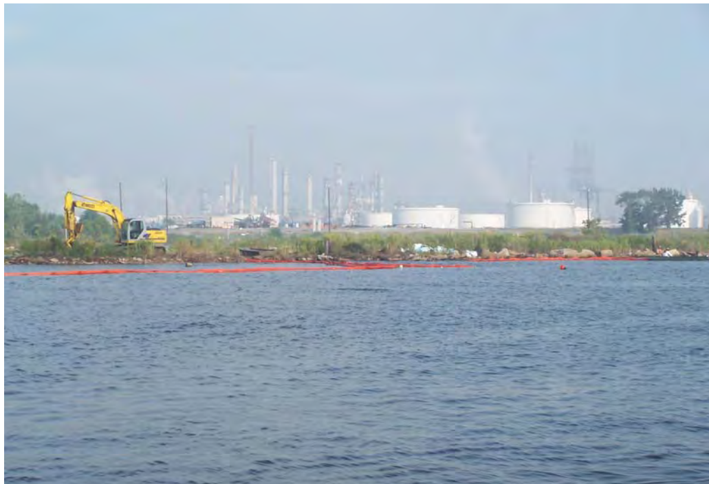
Photograph 10. View to northwest of CITGO facility with oil spill remediation activities in foreground.
