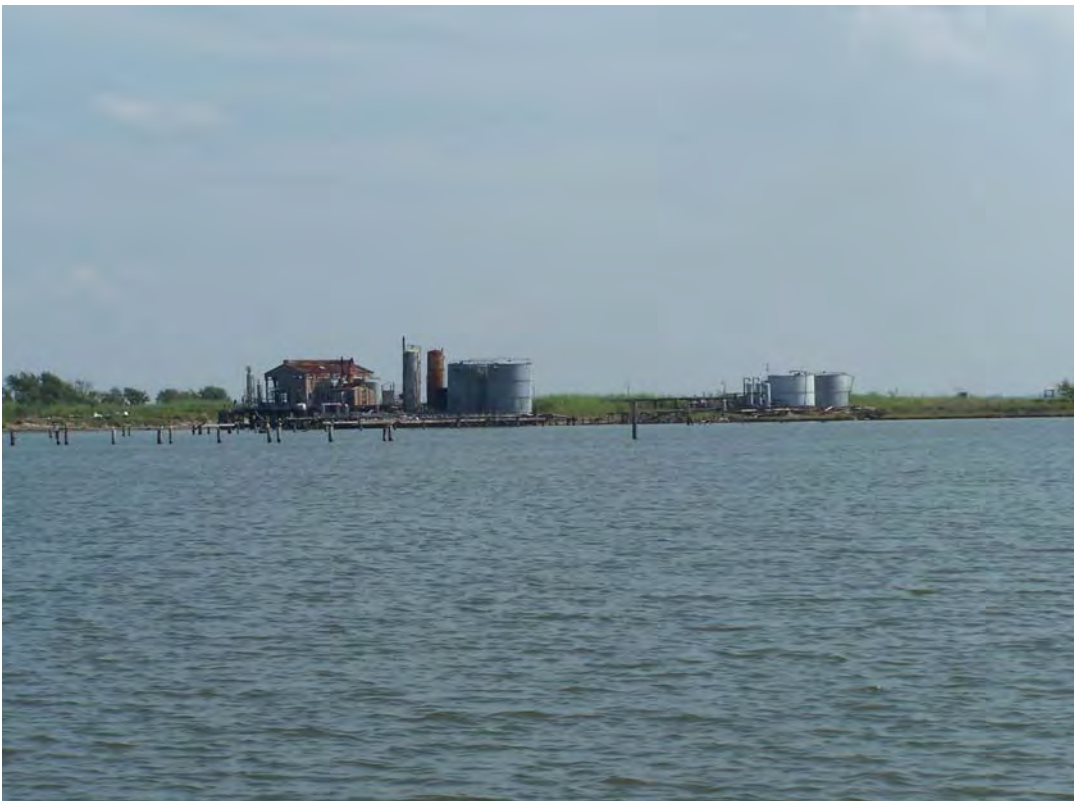
Photograph 28. View to east of East Hackberry Oil Field structures.
