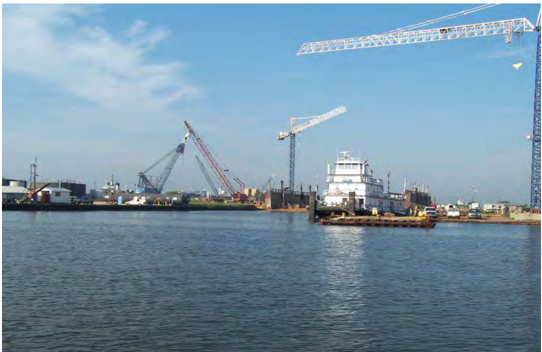
Photograph 19. View to north of Burtons Landing; note ASTs at center.
