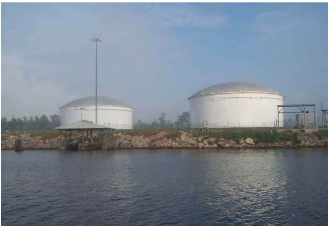
Photograph 8. View to northwest of LNG tanks at CITGO facility.
