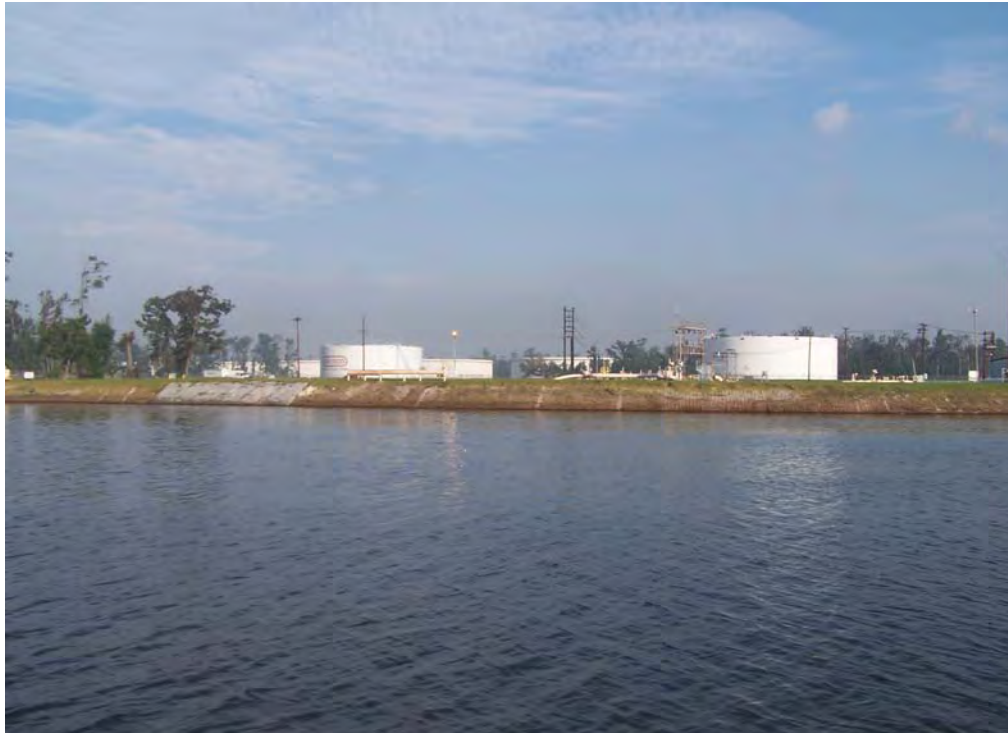
Photograph 13. View to west of Conoco Philips facility.
