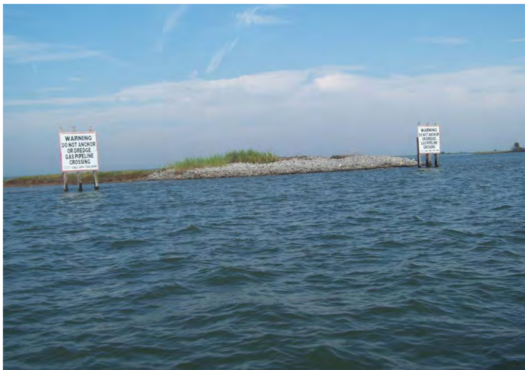
Photograph 36. View to northwest of pipeline crossing near north shore of West Cove.
