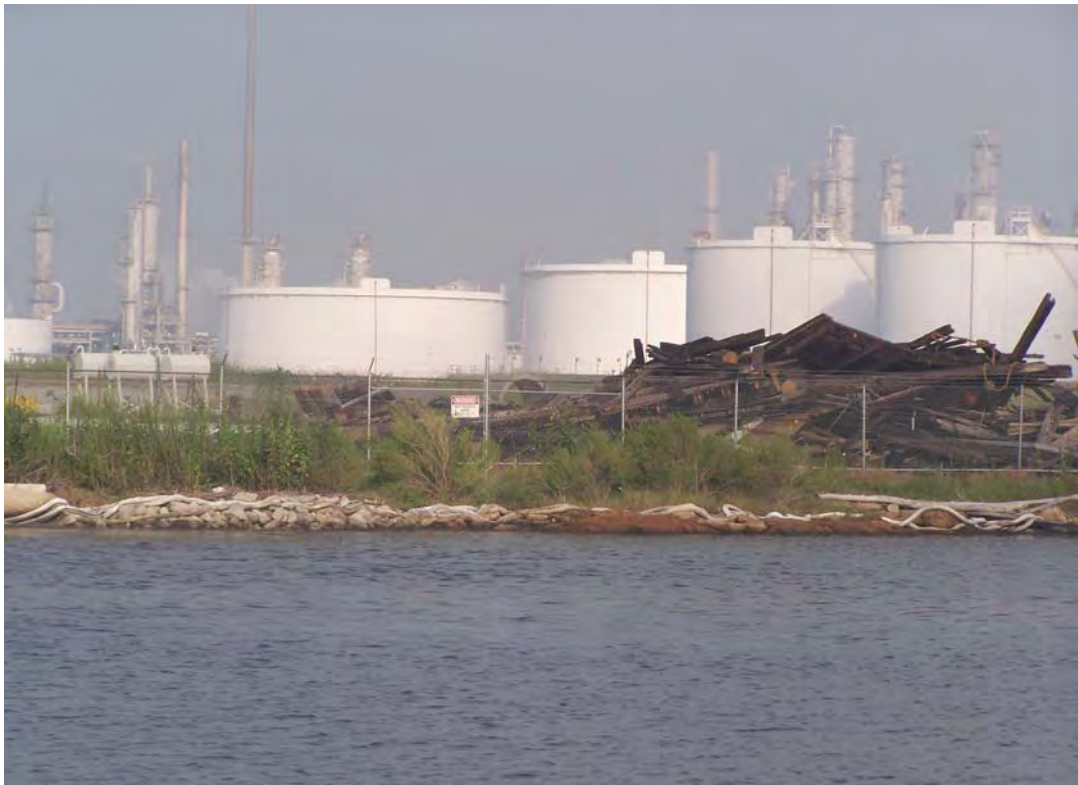
Photograph 9. View to northwest of CITGO facility with debris in foreground.
