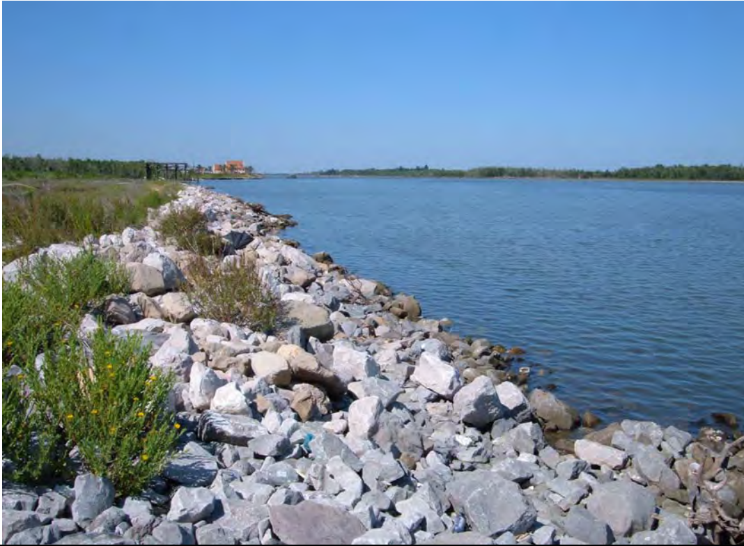
Photograph 25. View to north of west channel bank at Hackberry.
