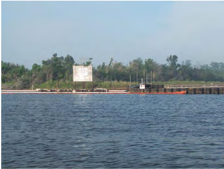
Photograph 11. View to west of pipeline crossing at CITGO facility with oil booms deployed.
