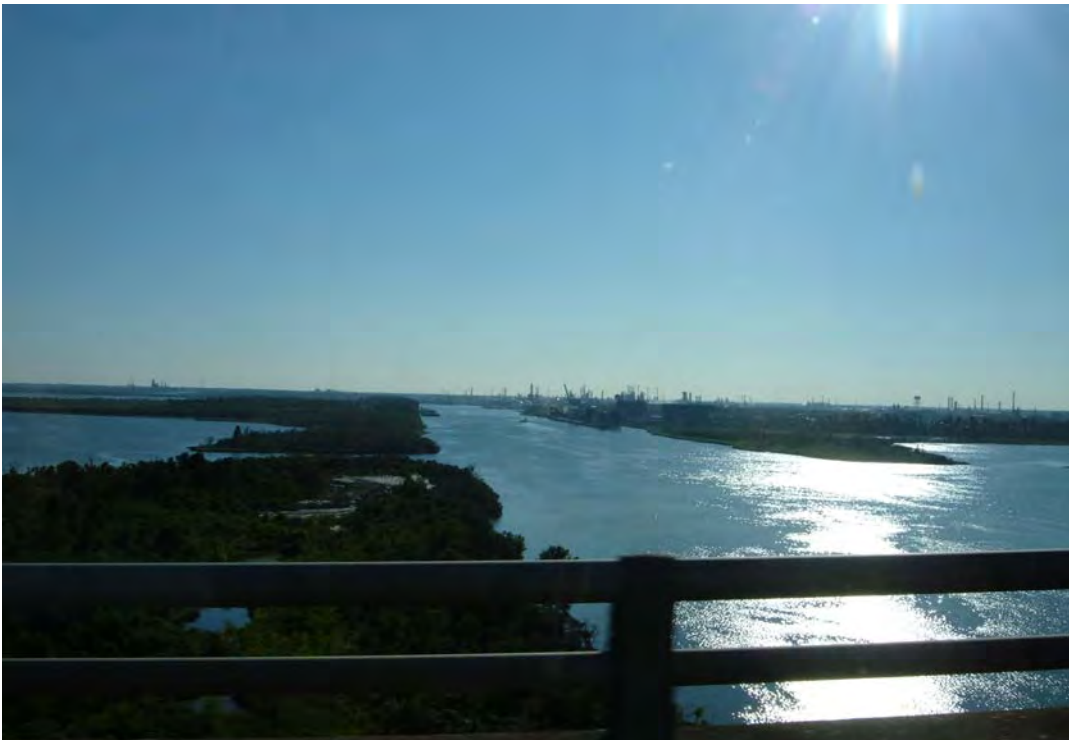
Photograph 3. View to south of channel from I-210 Bridge.
