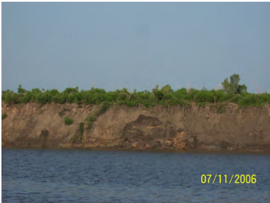
Picture 2 – Ship Channel View of Levee at PA 16S.
