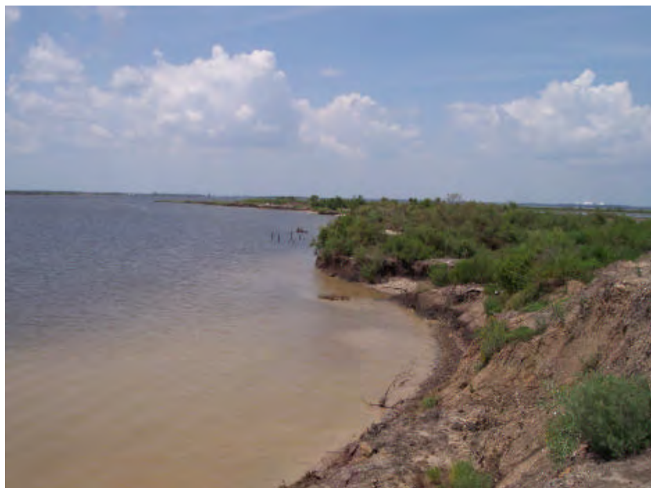
Picture 4 – North View of PA 17 along the Ship Channel.
