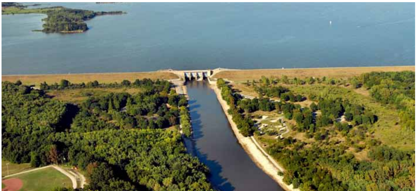
Aerial of the Carlyle Lake Dam. Photo by Allan Dooley.
