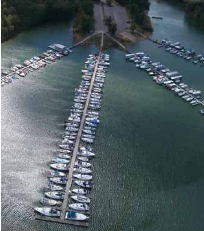
John H. Kerr Dam and Reservoir, Steel Creek Marina. U.S. Corps of Engineers photo by Joshua Davis.
