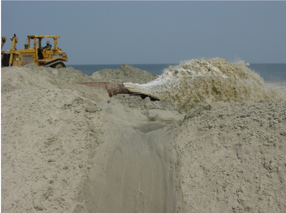
Figure 5.1. Example of beach fill being constructed (Masonboro Island, NC).
