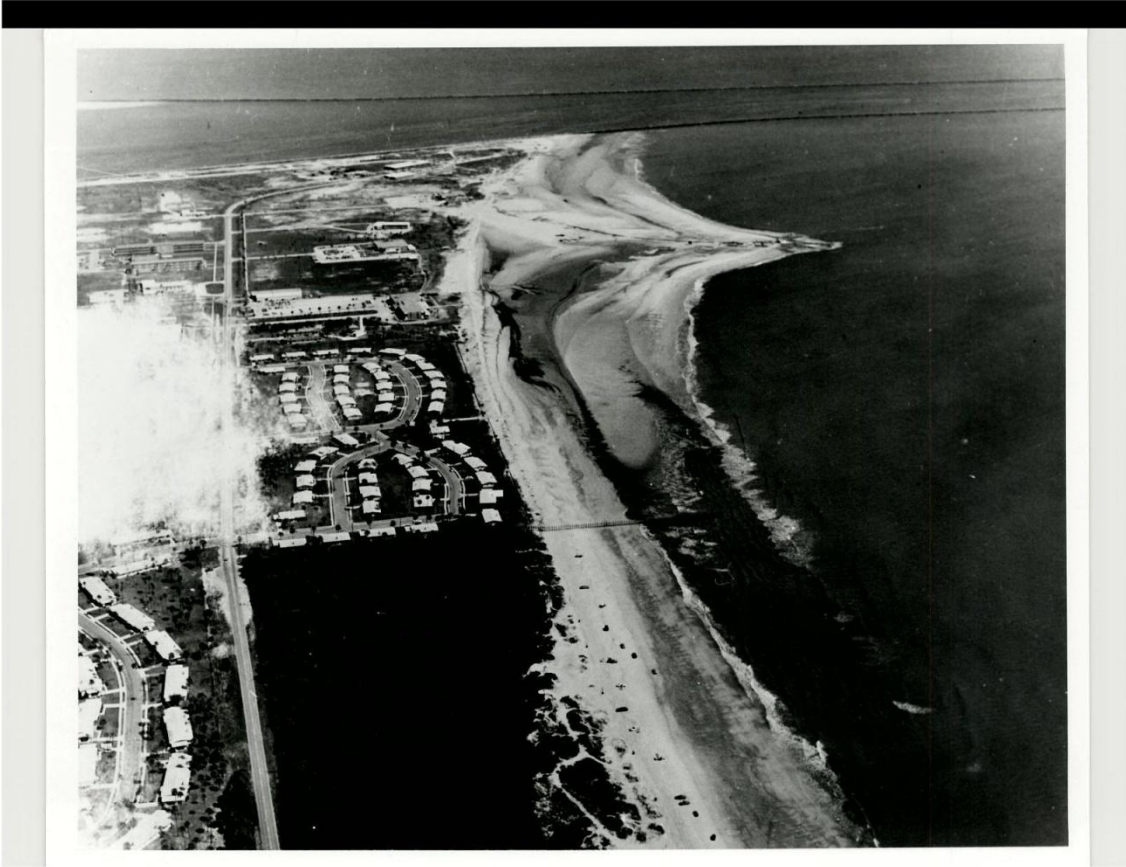
Figure 3: SAJ feeder beach construction near nodal point south of the St. Johns River entrance channel in 1972
