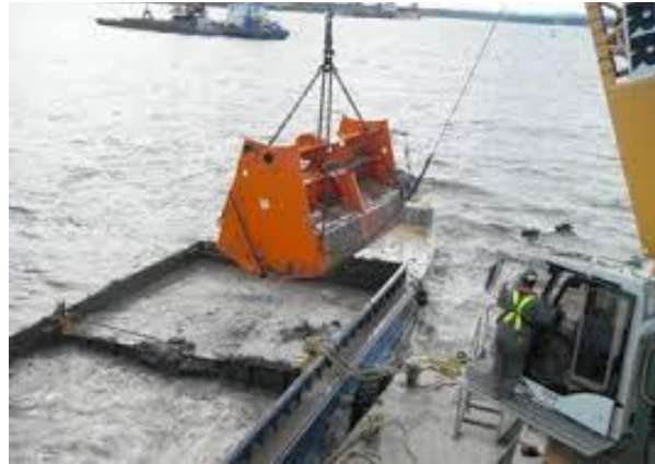
Loading a scow with via bucket operation.
