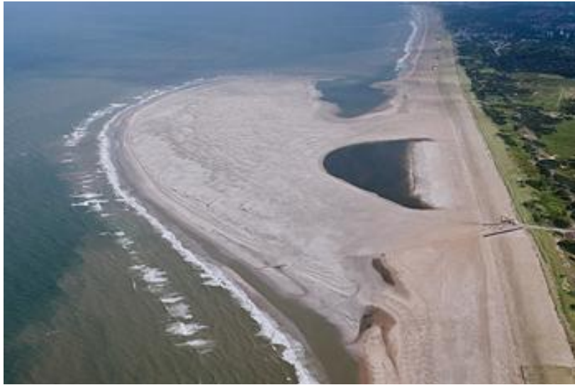
Figure 1: Feeder point (Sand Engine) construction in the Netherlands.
