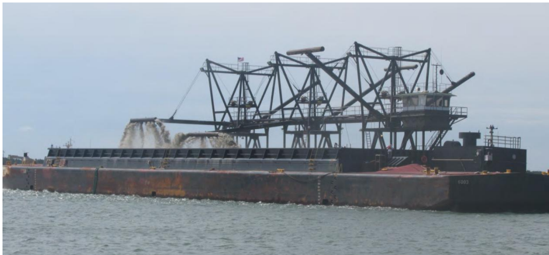
Hydraulic Cutter Head Dredge Loading a Scow Via Spider Barge
