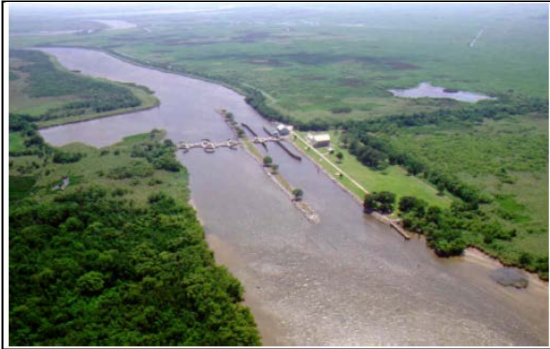
Photograph 1. Catfish Point Control Structure
