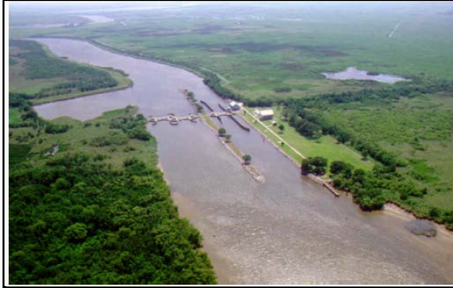
Photograph 1. Catfish Point Control Structure
