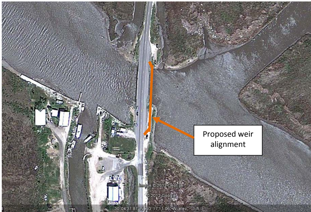
Sketch of the proposed alignment of the earthen-fill weir east of the existing culvert structure
