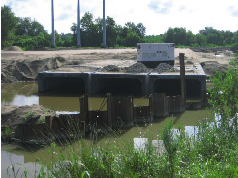
Pre-cast box culverts under construction – note the sheetpile cofferdam
