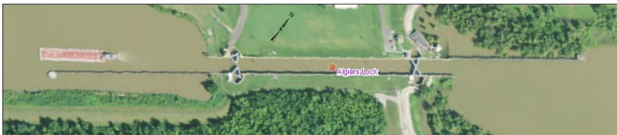
Figure A2- 50 Algiers Locks
