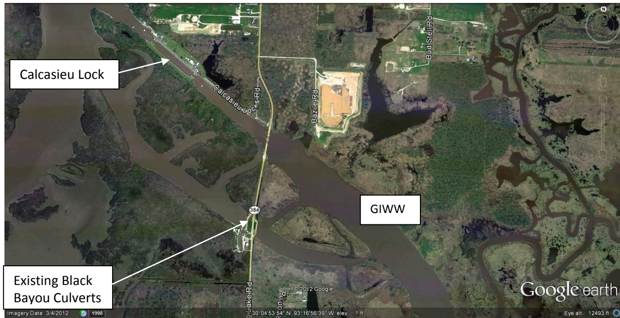
Existing conditions and relative location of Black Bayou Culvert structure to Calcasieu Lock Photo also shows the existing hydrologic connectivity of the area to the south of the Lock
