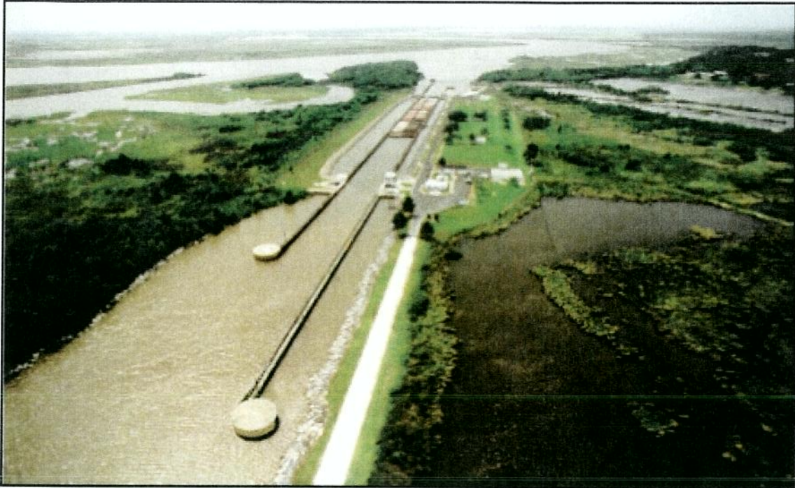
Calcasieu Lock Looking Northwest Toward Choupique Island and the Calcasieu River
