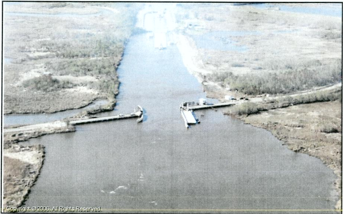
Calcasieu Lock and Pontoon Bridge Looking Southeast
