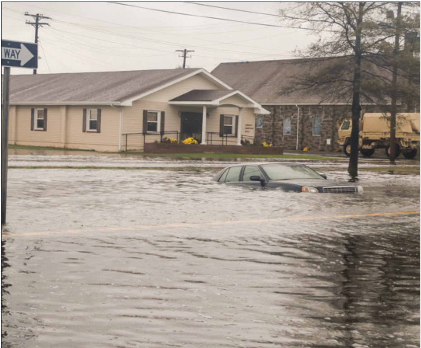
Hurricane Sandy flooding, Crisfield, MD on October 30, 2012
