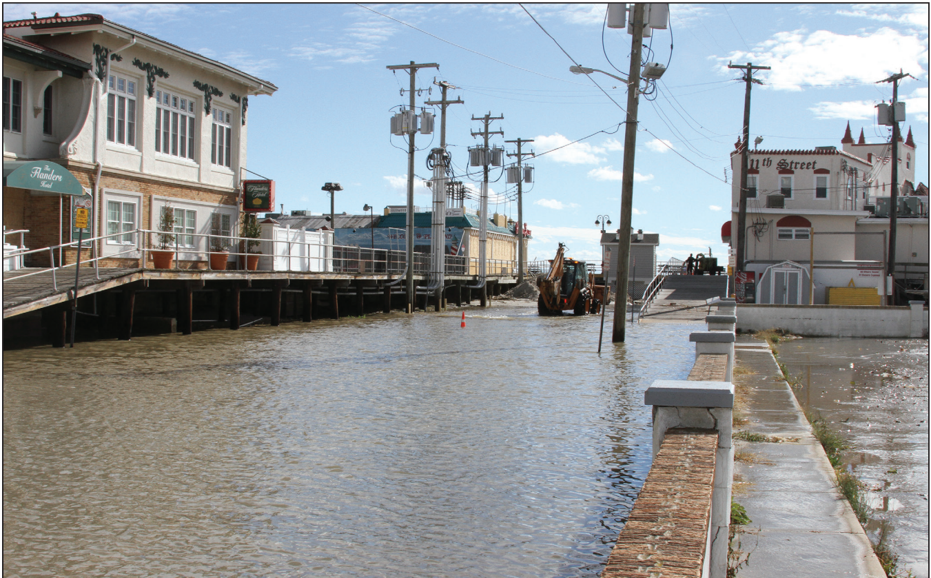
Flooding on 11th Street, Ocean City, NJ
