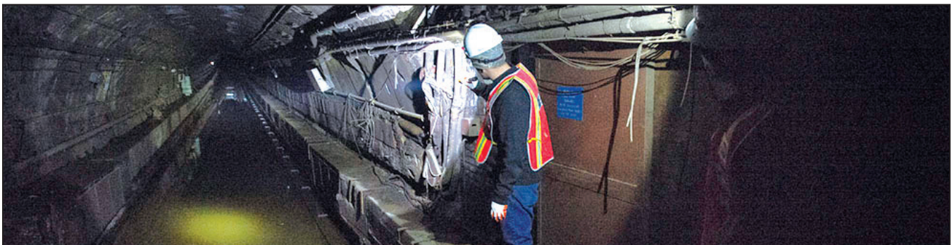
Metropolitan Transit Authority employees worked around the clock to remove seawater from a flooded subway tunnel in Manhattan, NY on November 5, 2012
