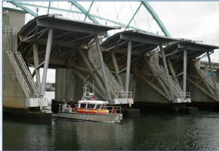
Figure II-1. Fox Point Storm Surge Barrier, Providence RI (Source: Providence Journal)
