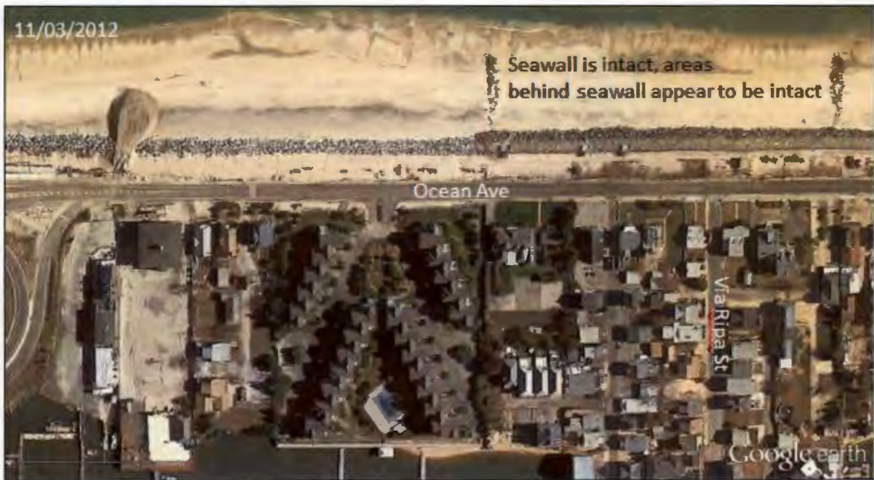
Figure 17: Post-storm beach condition at northern Sea Bright (area w/ seawall)
