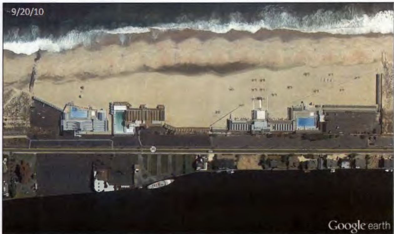
Figure 18: Pre-storm beach condition at Sea Bright (area w/o seawall)
