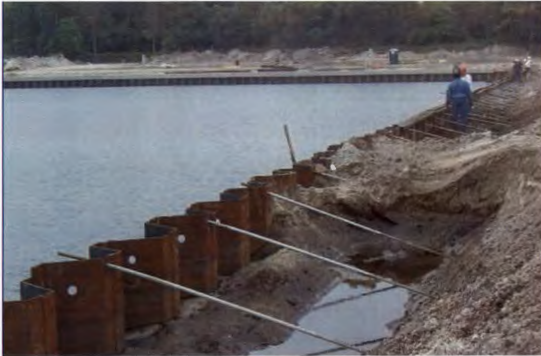
Figure D-8: Sheet Pile Bulkhead under Construction
