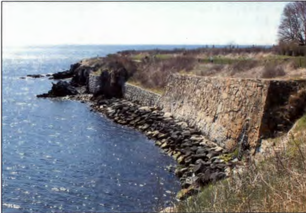
Figure D-7: Rock Revetment and retaining wall at Cliff Walk, Newport, RI
