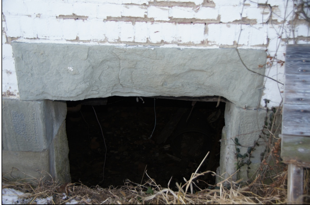
Photo 17. East foundation elevation showing former coal chute.
