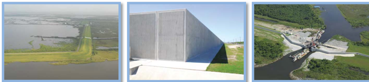
Figure 3-1: Typical levee, floodwall (T-wall) and control structure.
