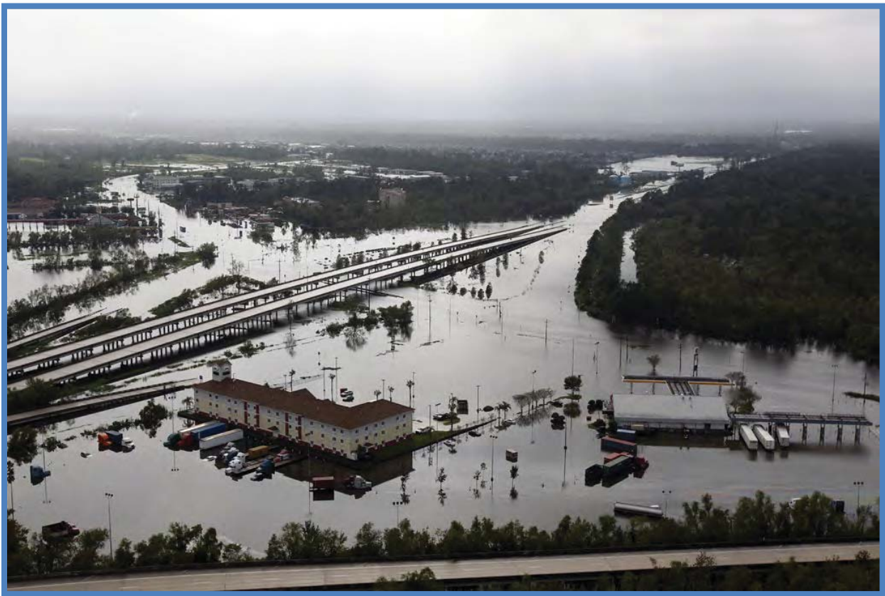
Hurricane Isaac flooding at I-10 and US-51.
