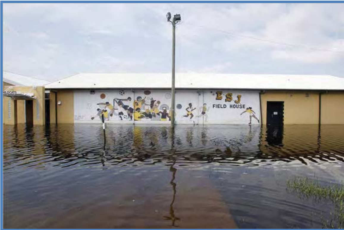
Figure 1-7: Hurricane Isaac flooding at East St. John High School. (Times-Picayune)
