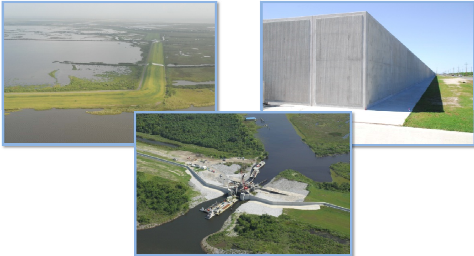
Figure 3-1: Typical levee, floodwall (T-wall) and control structure.
