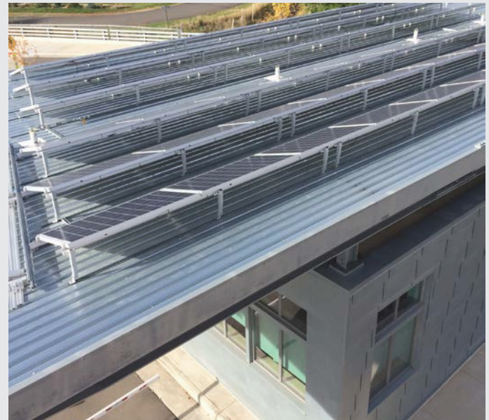
The SSEB at NREL had eleven new solar PV panels installed to bring the building back to a net zero energy status.
