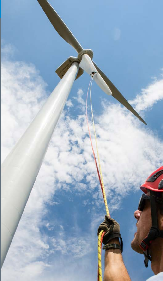
Pete Johnson (top) and Trask Bradbury with Gemini Rope Access Solutions work together as they inspect the blades of a 3MW Alstom turbine undergoing testing at NREL's National Wind Technology Center (NWTTC).
