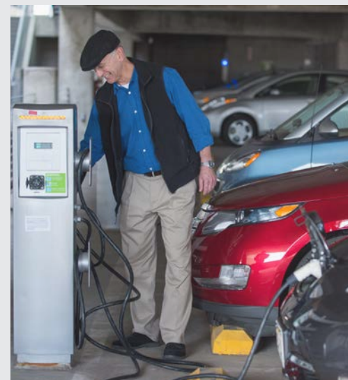
NREL employee Phil Pienkos charges his hybrid vehicle on one of the 36 electric vehicle charging stations in the NREL parking garage.
