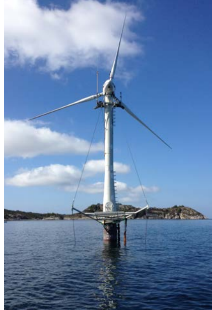
SWAY's one-fifth scale prototype demonstration wind energy system installed off the coast of Bergen, Norway. Photo by Eric Nelson, NREL/PIX 21966
