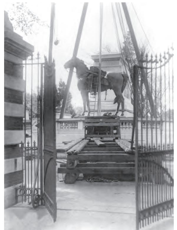
Designed by sculptor Henry M. Shrady, the central figure of the composition—the bronze equestrian statue of Grant—weighs 10,700 pounds and with its pedestal is forty feet high. The statue was hoisted atop its pedestal in 1919.
