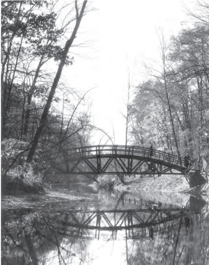
Timber footbridge over Rock Creek Park. This bowstring, or grapevine truss, bridge was located near Beach Drive and illustrates the rustic construction in the park.
