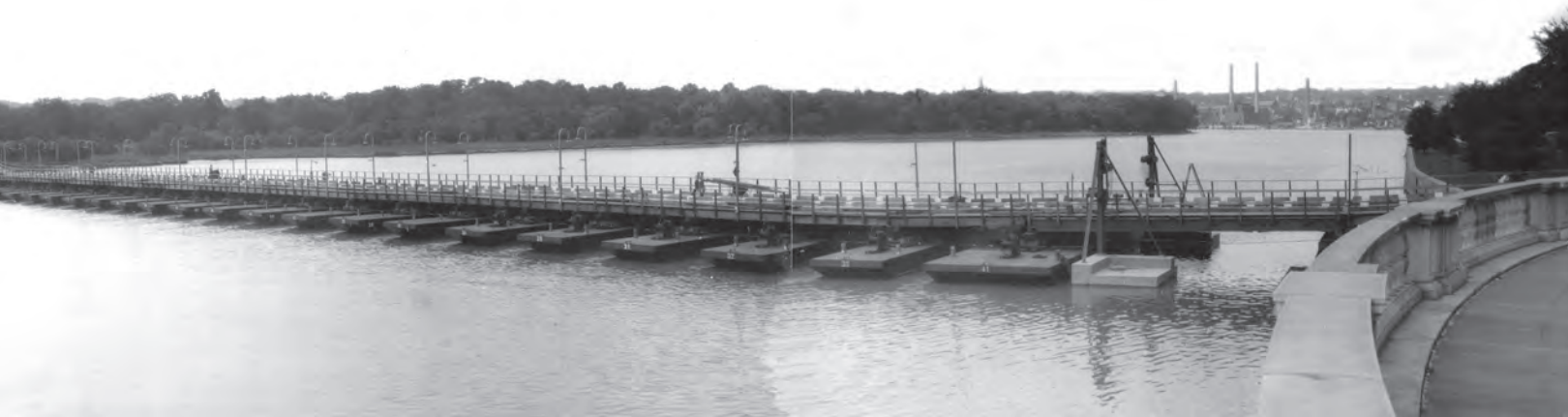
(Top) Emergency Railroad Bridge, August 1942. The Washington Engineer District built this additional, temporary crossing over the Potomac River from Shepherds Landing, D.C., to Alexandria, Virginia, to transport goods and troops in a national emergency. Authorities worried that the bridge immediately to the north was the only rail crossing of the southern Potomac River. National Archives no. 77-RH-141B-1
