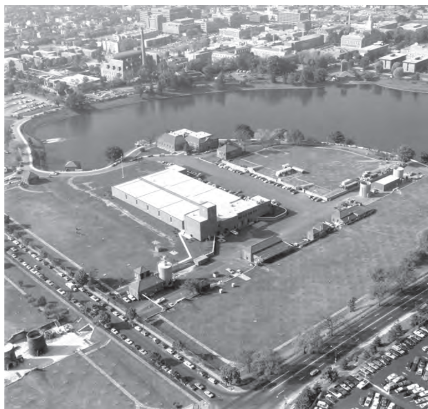
Beginning in 1982 the construction of new rapid sand filters at the McMillan reservoir, just east of Howard University, obviated the need for the slow sand filters built in 1905. The sand storage “silos” (extreme lower left) remained standing in 2004 as remnants of the earlier technology. Washington Aqueduct Division, Baltimore Engineer District
