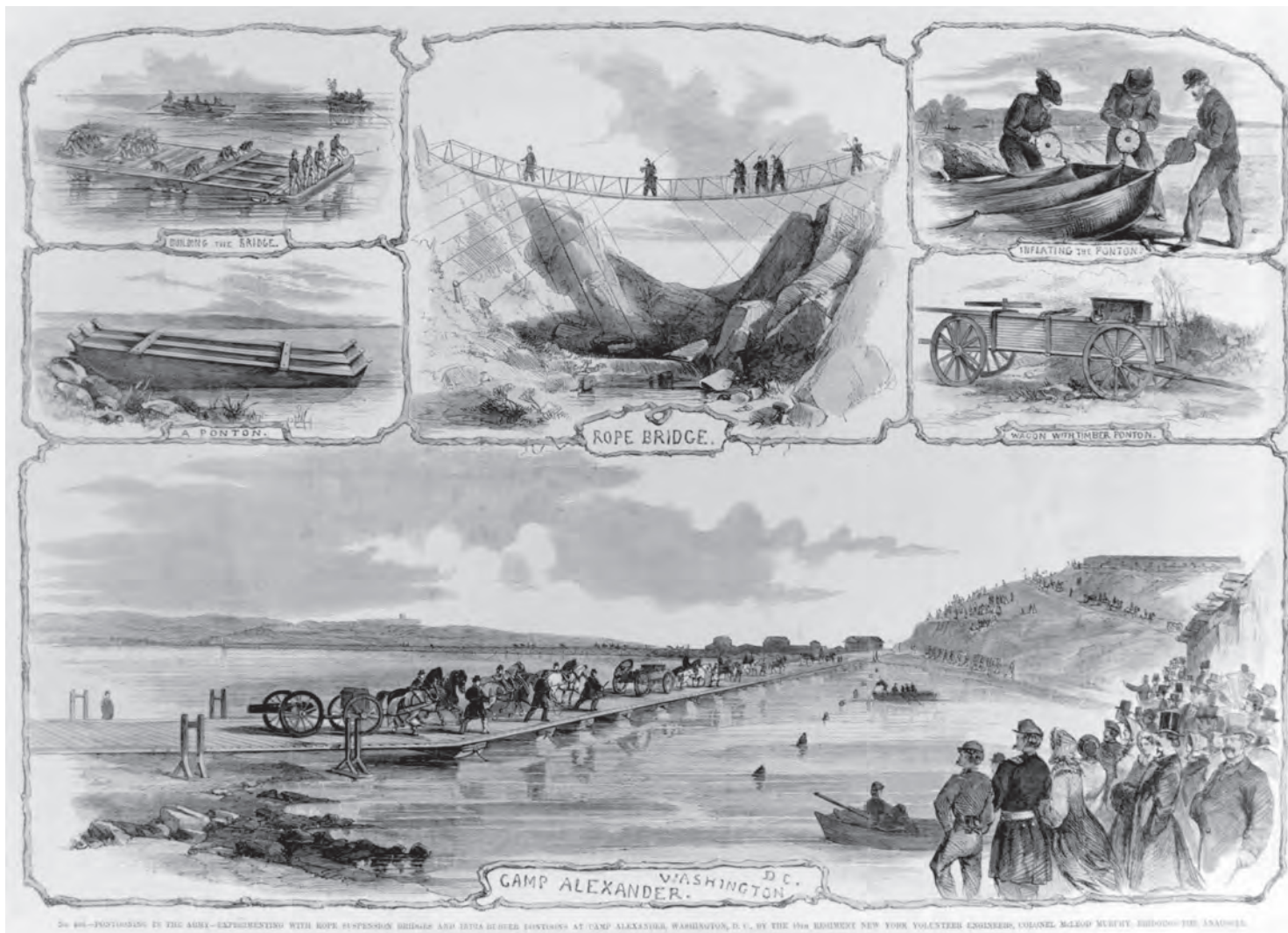
Lithograph of the 15th New York Volunteer Engineers experimenting with rope suspension bridges and India rubber pontoons and ponton bridges at Camp Alexander on the Anacostia River during the Civil War Office of History, Corps of Engineers
