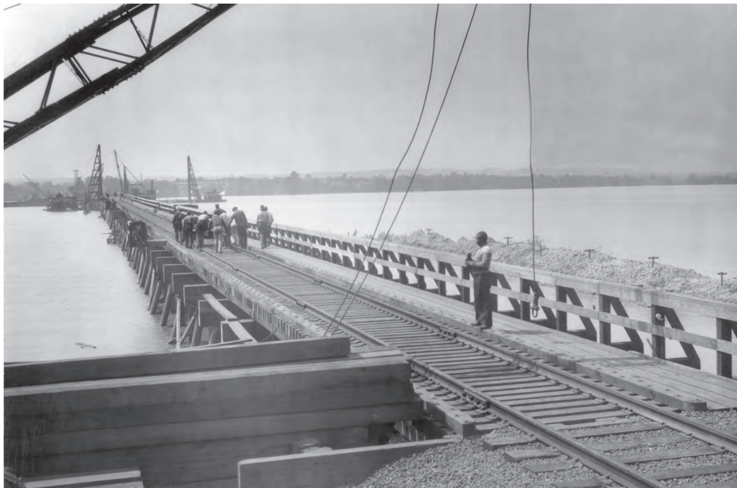
(Top) Emergency Railroad Bridge, August 1942. The Washington Engineer District built this additional, temporary crossing over the Potomac River from Shepherds Landing, D.C., to Alexandria, Virginia, to transport goods and troops in a national emergency. Authorities worried that the bridge immediately to the north was the only rail crossing of the southern Potomac River. National Archives no. 77-RH-141B-1
