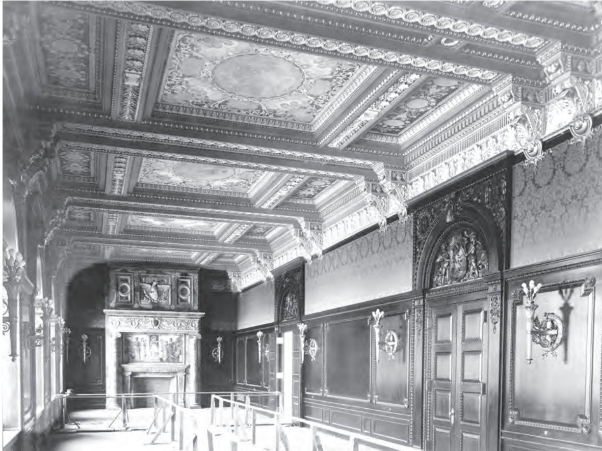
Private reading room, House of Representatives, under construction, designed by Edward P. Casey
