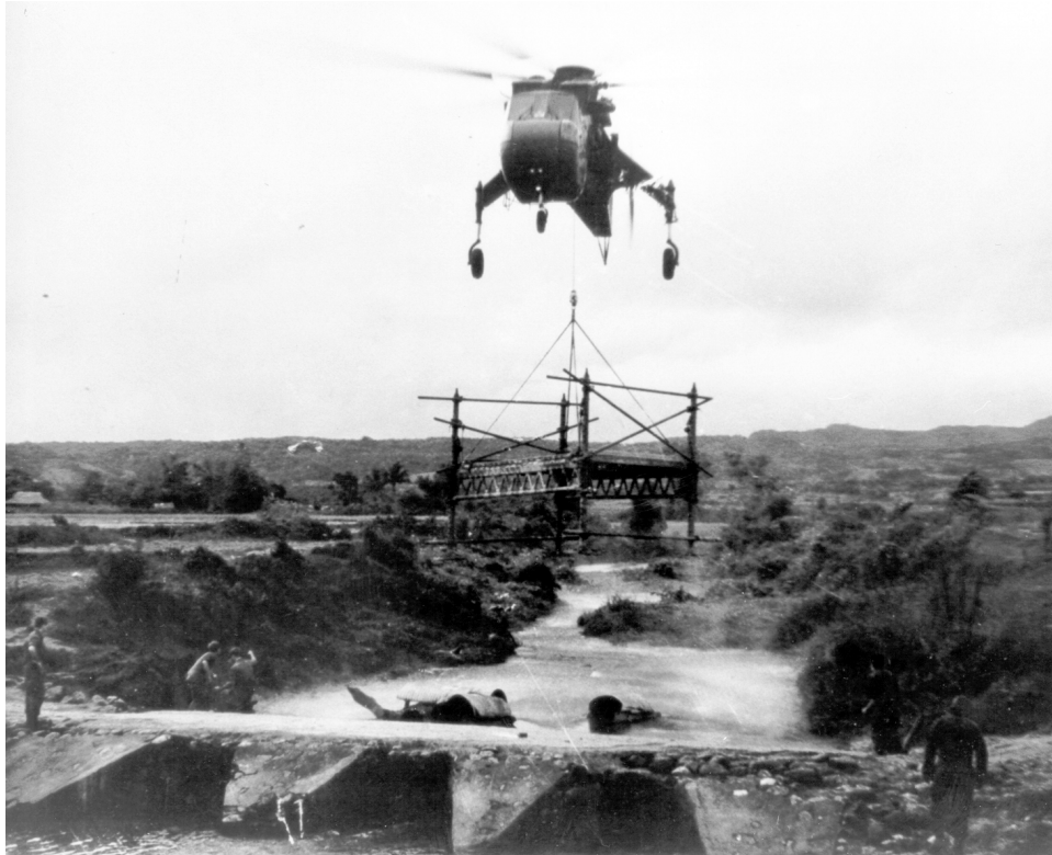
U.S. Army helicopters leapfrogged M4T6 trestles along the route from Tuy Hoa to Cung Son in February 1969.
