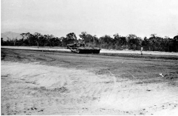
In May 1962 Company B of the 201st Engineer Battalion was rebuilding the French airfield at An Khe.
