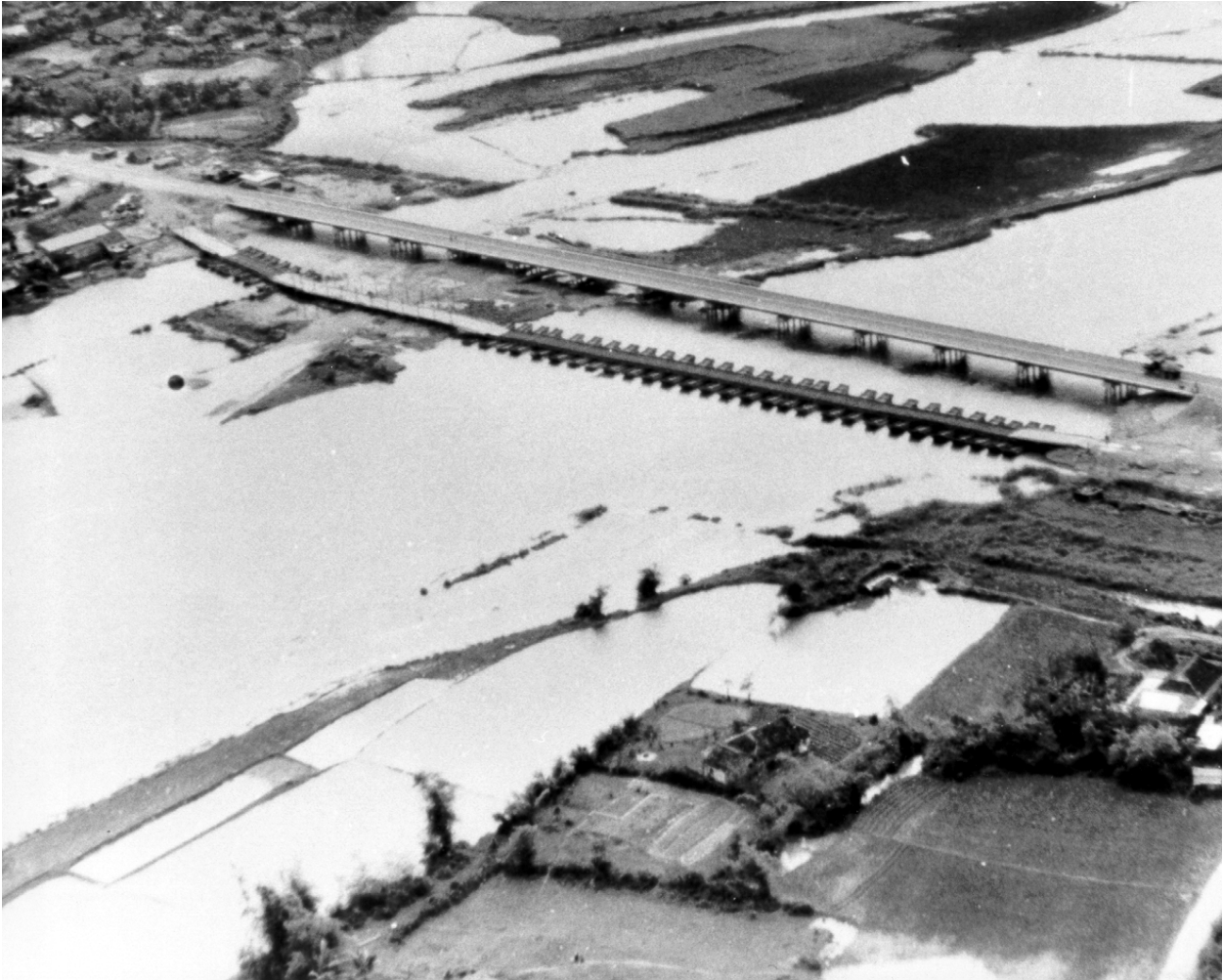
Army Engineer bridges over the Ban Thach River in South Vietnam. In the foreground was an M4T6 bridge and the background an 840-foot, 13-pier bridge.
