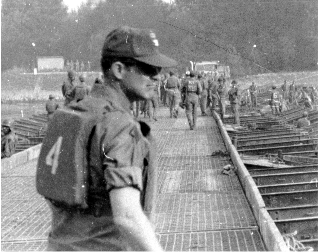
Colonel Kem inspected the bridging exercises on the Rhine River conducted by the labor service companies and the 565th Engineer Battalion in the spring of 1977.
