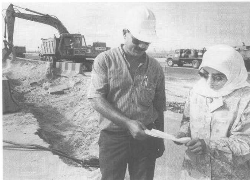
A Corps contractor and Kuwaiti volunteer discuss road repair.
