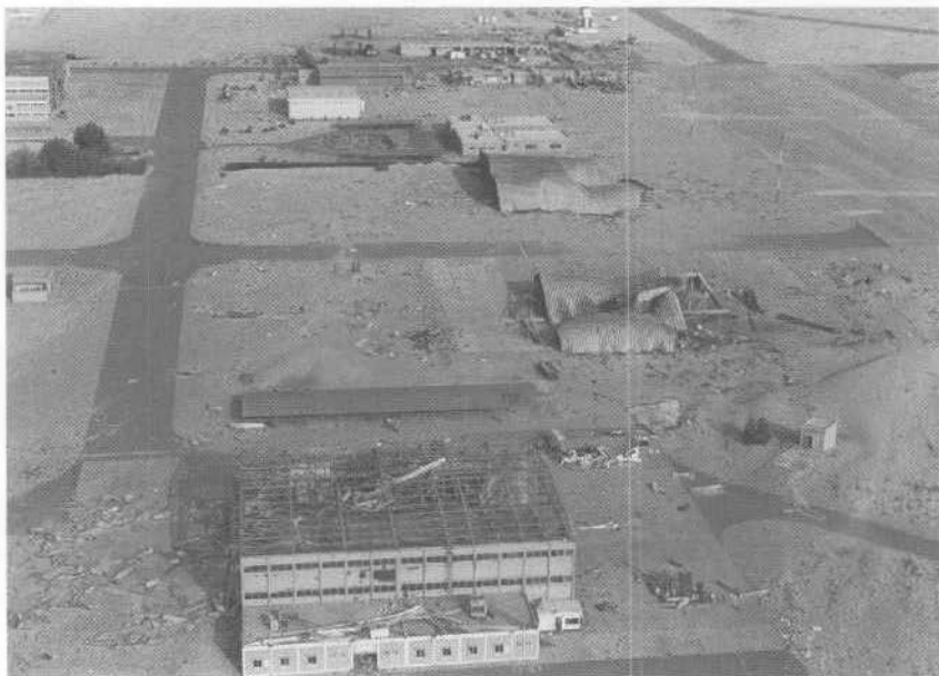
Aerial view of the damage to Ahmed Al-Jaber Air Base
