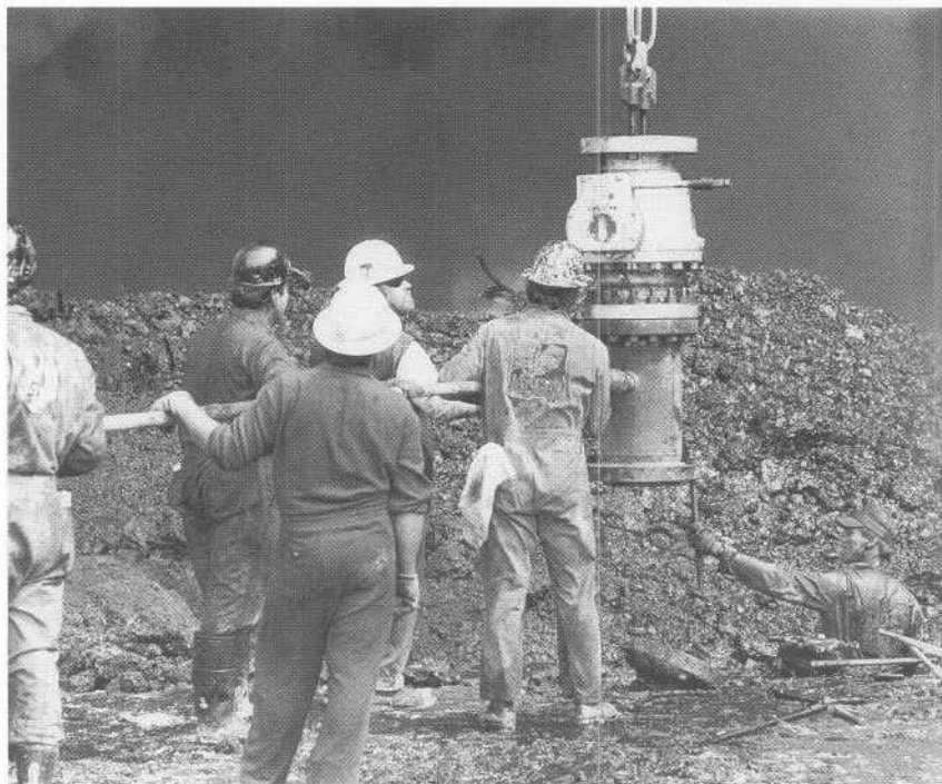
Oil well firefighters cap an oil well.
