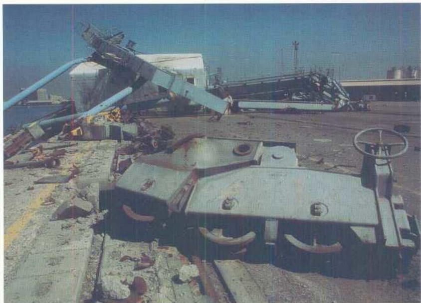
Facilities at Shuwaikh port were badly damaged.
