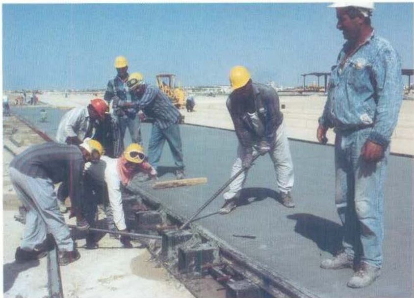
Repair work at Al-Jaber Air Base
