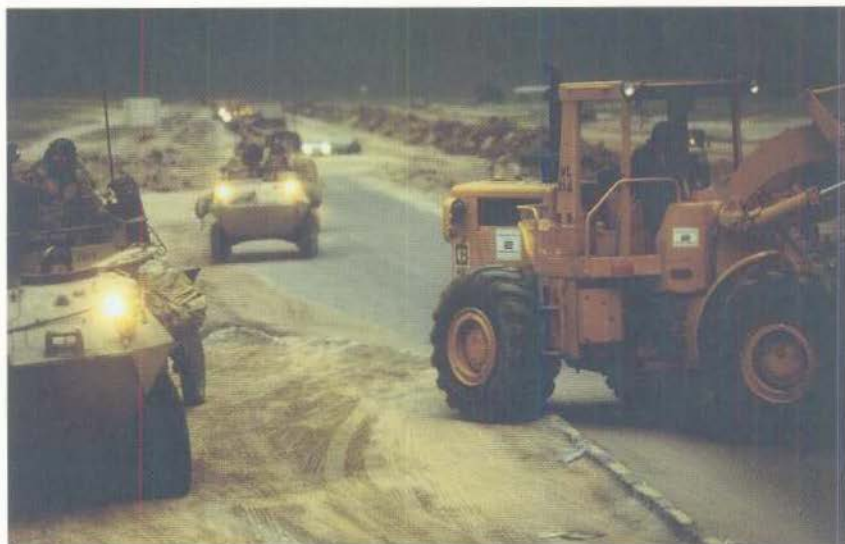
Power cable repair south of Kuwait City
