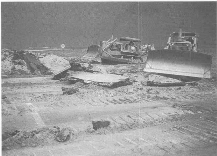
Contractors repair roads in Kuwait.
