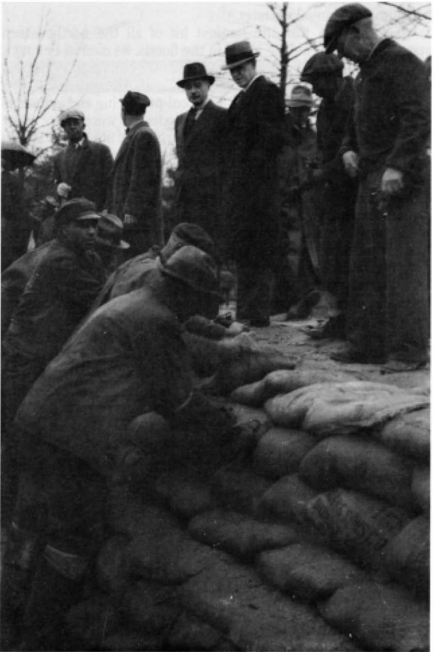
Engineer Lieutenant Colonel Francis C. Hawington (above, left center) with the Works Progress Administration, and Harry L. Hopkins (right center), Administrator of the WPA, watching workmen erect an emergency levee in rear of Munitions Building, Washington, DC, March 1936.
