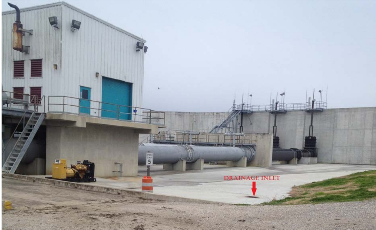
Figure 4: Proposed location of safe house on protected west side of St. Mary Pump Station on an existing concrete slab and possible relocation of drainage inlet
