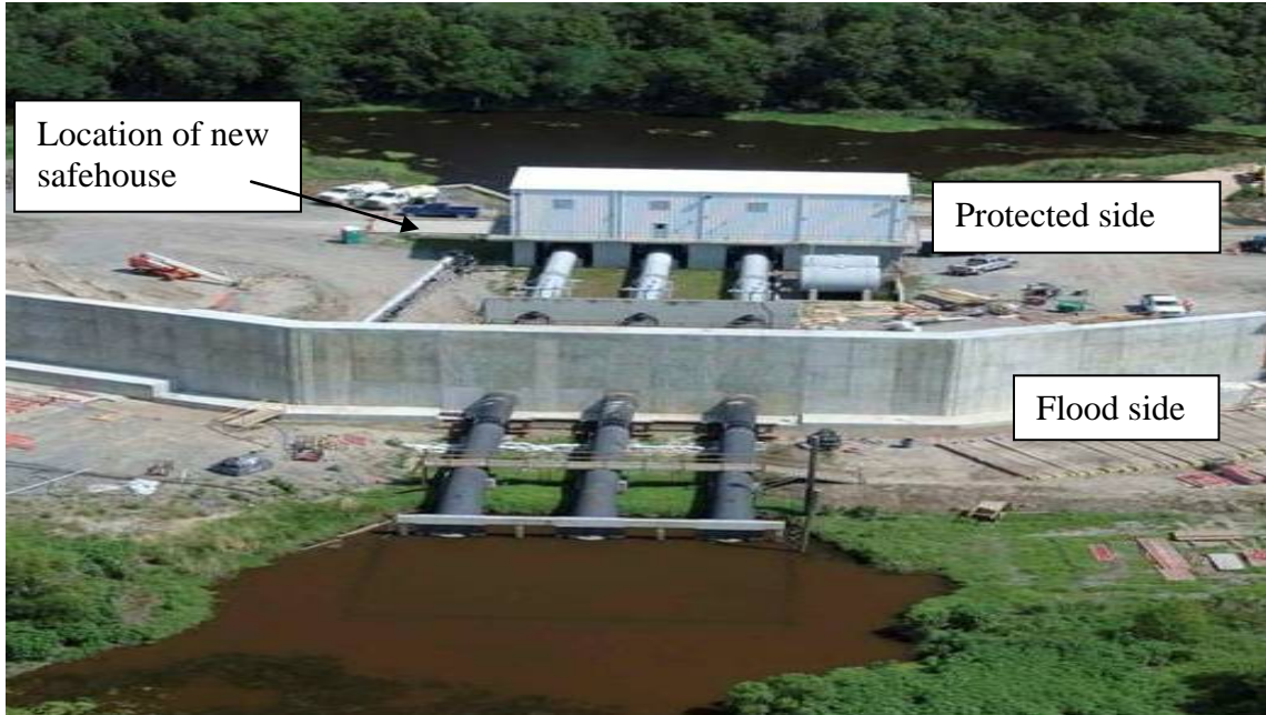
Figure 2 – St. Mary’s Pump Station during construction of the LPV 148.02A floodwall
