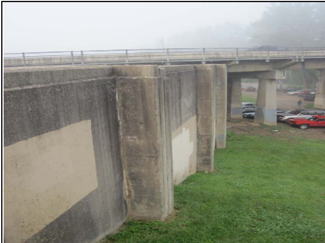
Figure 3: Three external waterstop pilasters on riverside of Newport, KY floodwall
