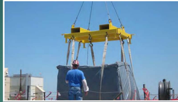
W.R. Grace Building 23 Remediation
