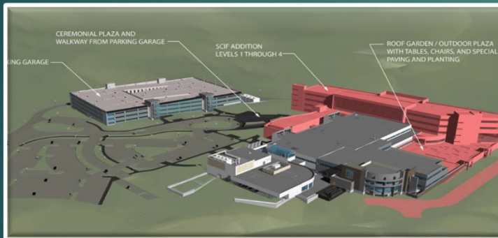
Ft. Belvoir Sensitive Compartmented Information Facility
