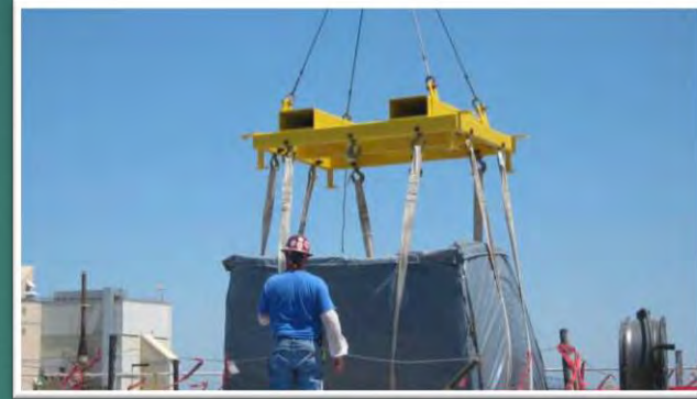
W.R. Grace Building 23 Remediation
