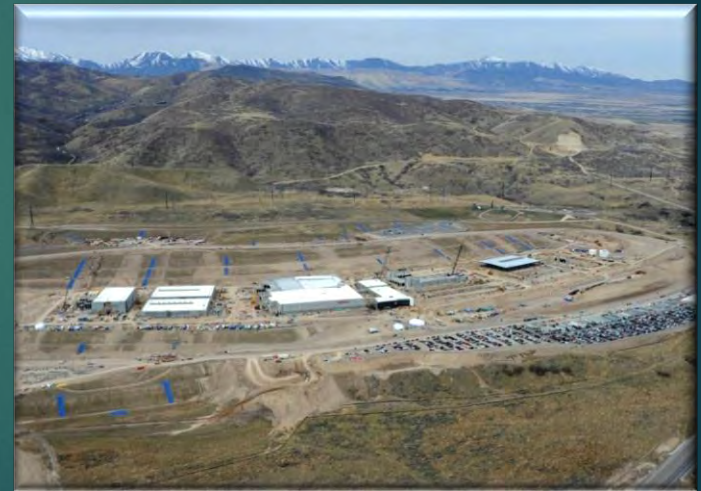
Utah Data Center
