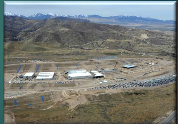
Utah Data Center
