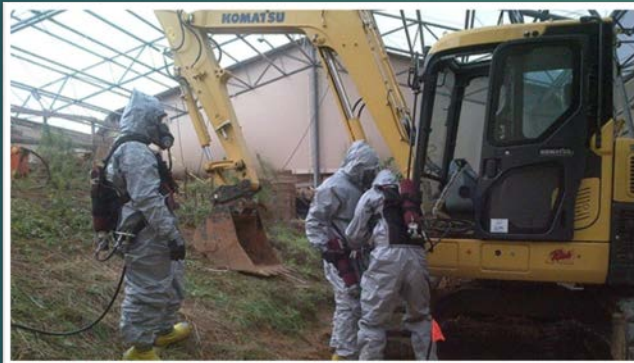
Spring Valley Formerly Used Defense Site
