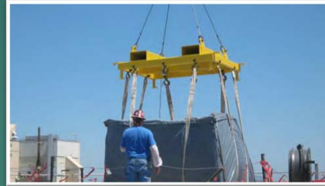
W.R. Grace Building 23 Remediation
