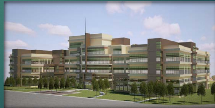
Replace DLA Headquarters, New Cumberland, PA, FY12
