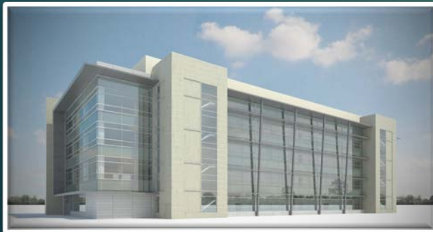
East Campus Building Marine Corps
