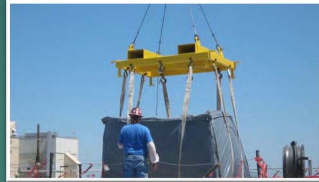
W.R. Grace Building 23 Remediation
