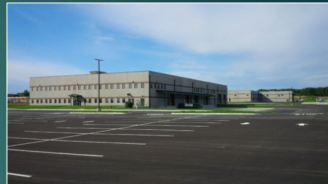
Consolidated Logistics Facility, Ft Detrick
