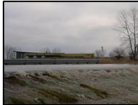
Flooding winter 2015 caused damages to project areas as well as shoaling in navigation channel leading to increased dredging costs
