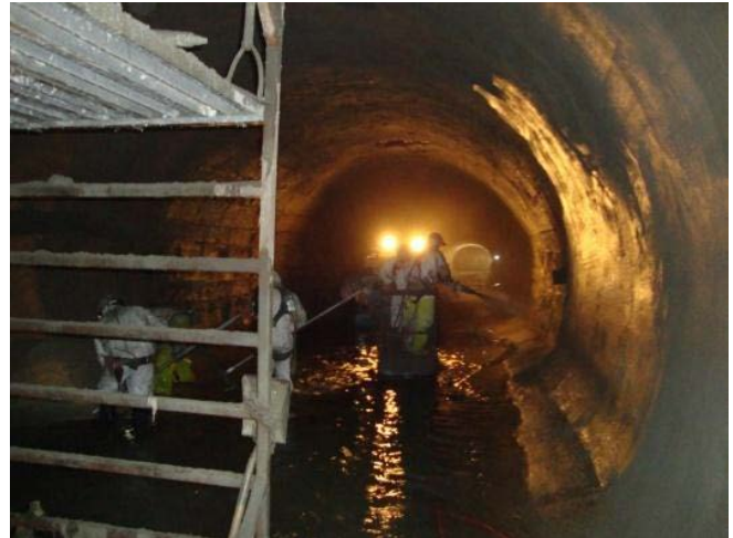
Old Mill Creek Sewer Line Repairs
