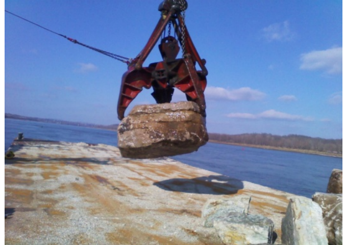
Figure 1. Rock Removal near Thebes, IL
