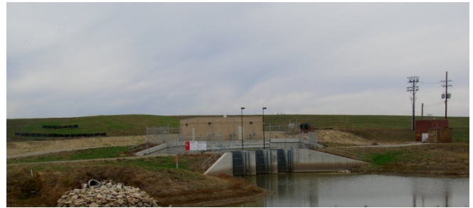
New Chain of Rocks Pump Station
