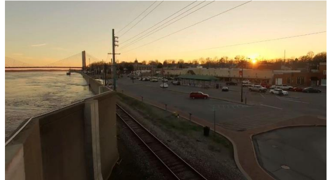
Cape Girardeau Floodwall
