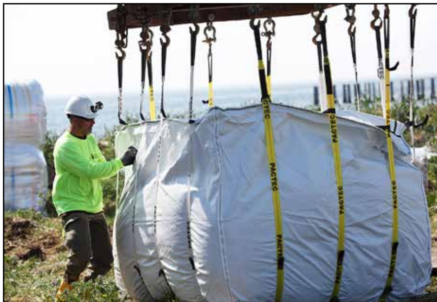
John Mura, an unexploded ordnance technician for Bristol Environmental Remediation Services, LLC, secures a load of contaminated soil before it is taken to a staging area, where it will be shipped out by barge in the fall to a permitted disposal facility in the Lower 48.
