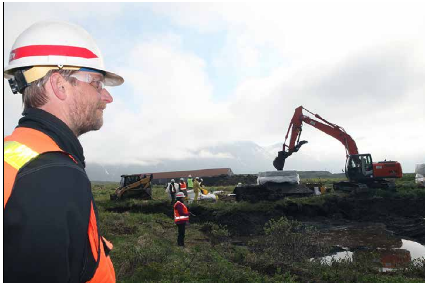
Andy Sorum, project manager with the Formerly Used Defense Sites program, U.S. Army Corps of Engineers, Alaska District, looks on as employees with Bristol Environmental Remediation Services, LLC, load and prepare to bag contaminated soil June 20 during an environmental cleanup project at Attu Island.
