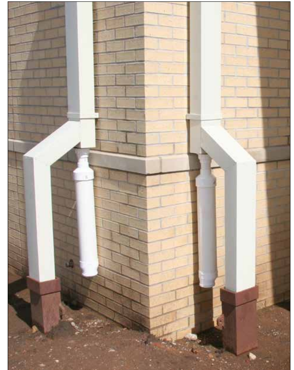
ABOVE: The 30,000-gallon rainwater collection tank at the Reception Complex under construction at Fort Sill. RIGHT: The first flush filter system in place at the Thermal High Altitude Air Defense project. BELOW: A look at the Mission Training Complex where photovoltaic panels are in place on the roof, just visible above the HVAC units. (Photos by Brant Purdum, Tulsa District)
