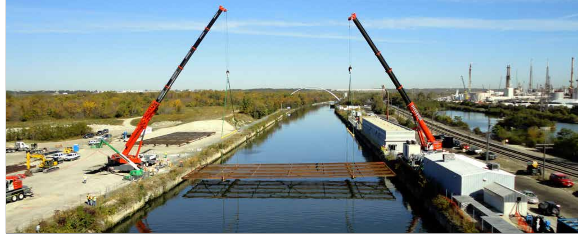
Underwater structures, known as parasitics, are placed into the Chicago Sanitary and Ship Canal as part of the electric barriers project in October 2010. The electric barriers deter the inter-basin establishment of Asian carp and other fish through an electric field in the water. Huntsville Center helps Army Corps of Engineers facilities like Chicago District's electric fish barriers — which are already using the best technology available for their specific operation — to find alternatives for reducing energy consumption. (Photo by Sarah Gross, Chicago District)
