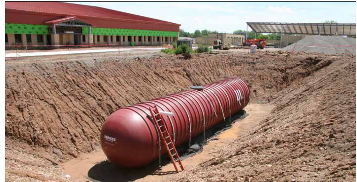
ABOVE: The 30,000-gallon rainwater collection tank at the Reception Complex under construction at Fort Sill. RIGHT: The first flush filter system in place at the Thermal High Altitude Air Defense project. BELOW: A look at the Mission Training Complex where photovoltaic panels are in place on the roof, just visible above the HVAC units. (Photos by Brant Purdum, Tulsa District)
