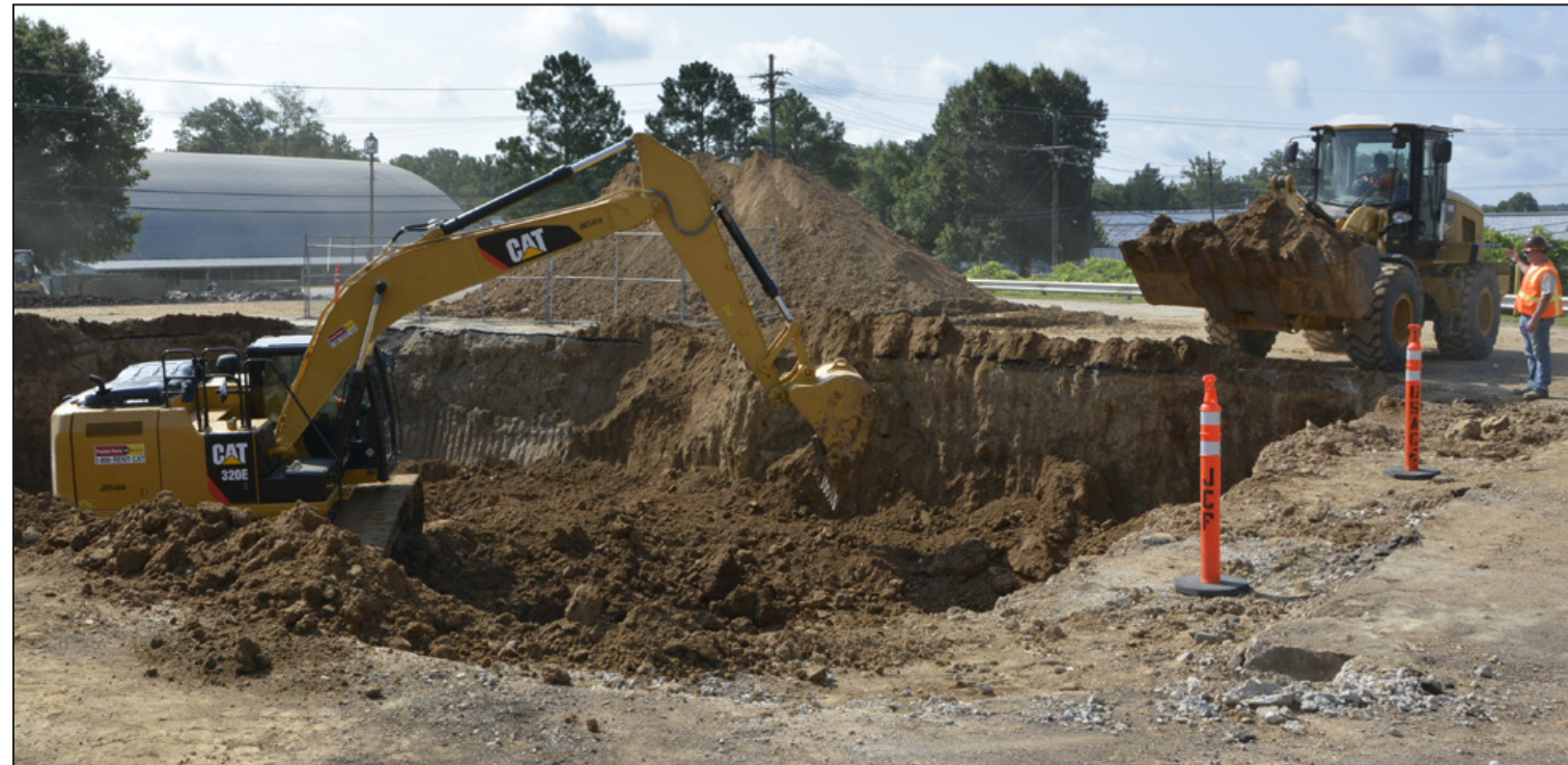
Some 2,500 cubic yards of soil were excavated, treated for contaminants and replaced during cleanup of a former motor pool site at the U.S. Army Engineer Research and Development Center in Vicksburg, Mississippi. The Vapor Energy Generator soil remediation system was used for the project, coordinated by the Omaha District. (Photo by Kerry Larsen)
