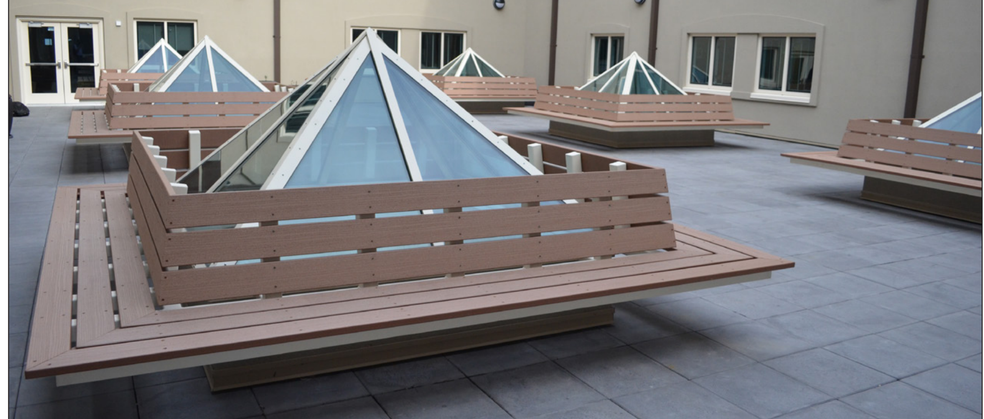
The interior courtyard of the new general instruction building for the Defense Language Institute Foreign Language Center at the Presidio of Monterey in California Oct. 16. The skylights are designed to provide natural light to the conference room below it, cutting electricity costs. The building incorporates the latest energy and water conservation technologies in order to operate more efficiently and in a sustainable, environmentally friendly manner.
