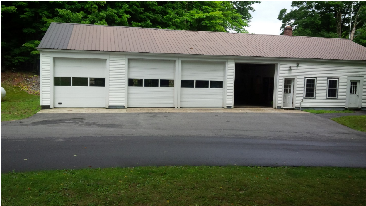
Informational Photo Number 1: Surry Mountain Lake – Current condition of apron
